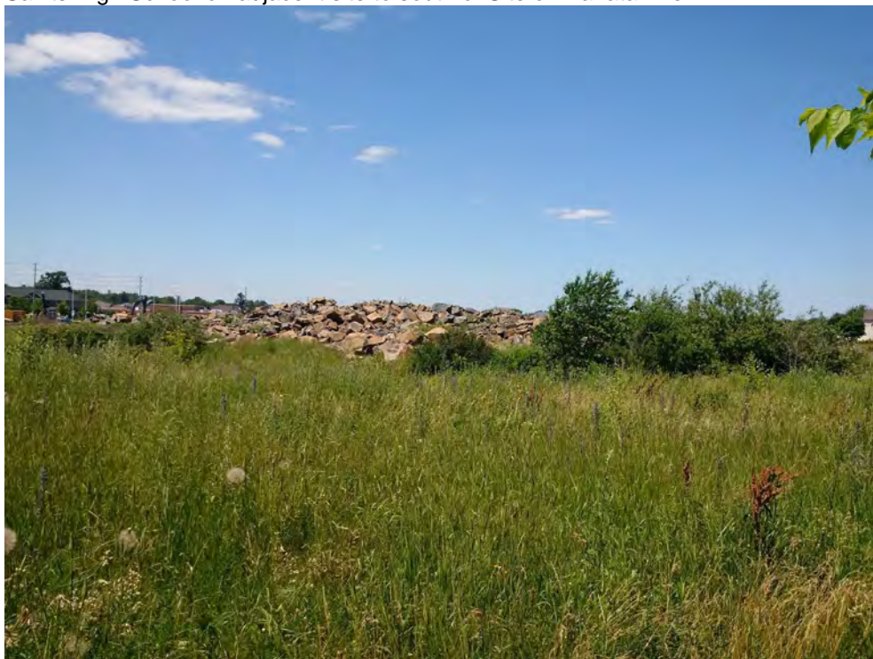
Photo 6: View of south site of Site looking north.
