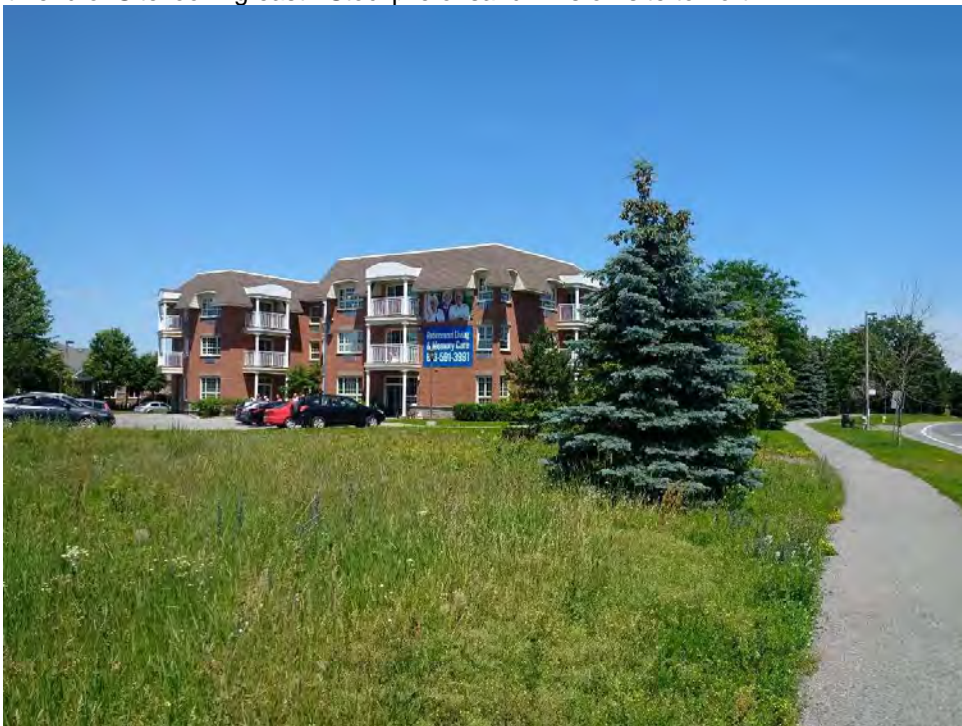
Photo 4: Southeast corner of Site on Kanata Ave, looking east at adjacent Senior's Residence.
