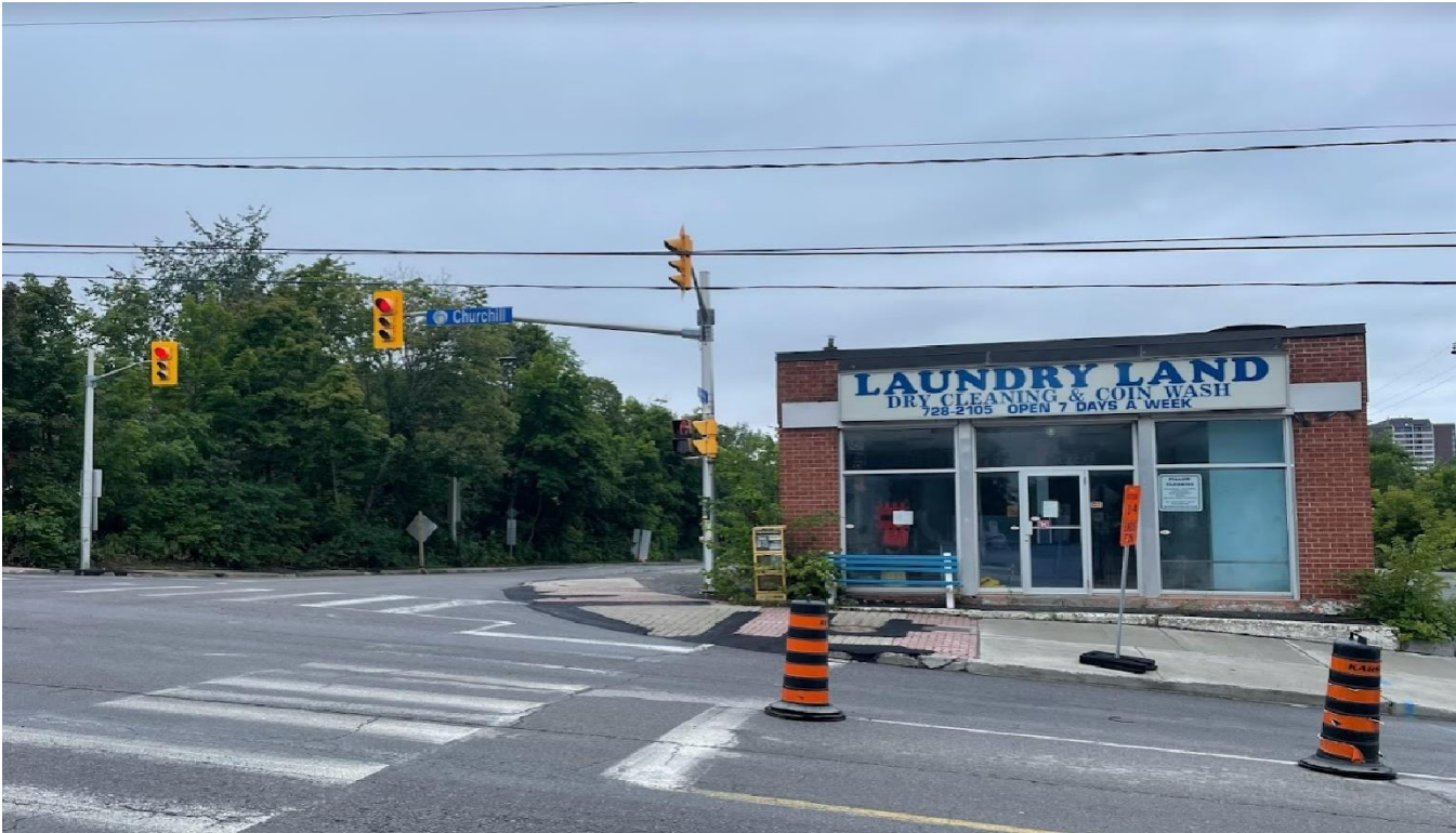
Figure 5: Subject site, looking west at Churchill Avenue North and Byron Avenue intersection
