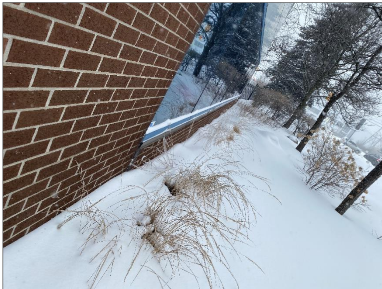
Photo 4 – Site Building (partial view of the north elevation).
