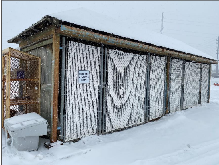
Photo 11 – Former Coal Tar Storage Shed.
