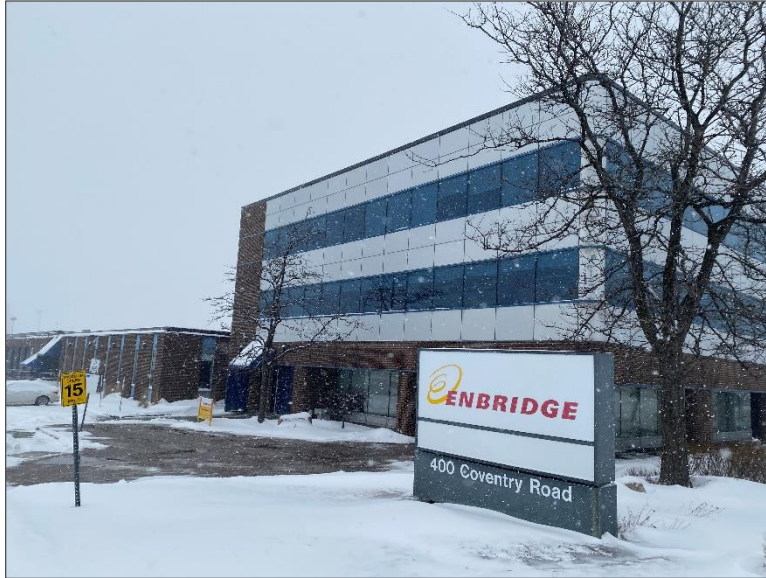
Photo 1 – Site Building (south elevation).
