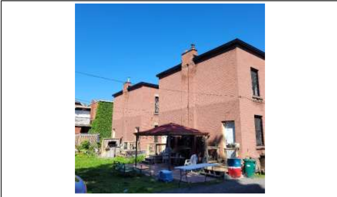
Photograph 25: Looking north-west from south-east end of 18 Hawthorne at back (south end) of buildings.
