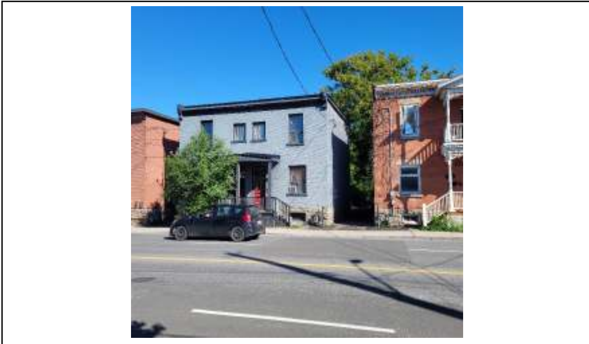
Photograph 31: Looking north from 18 across Hawthorne Avenue towards residential buildings on Hawthorne.
