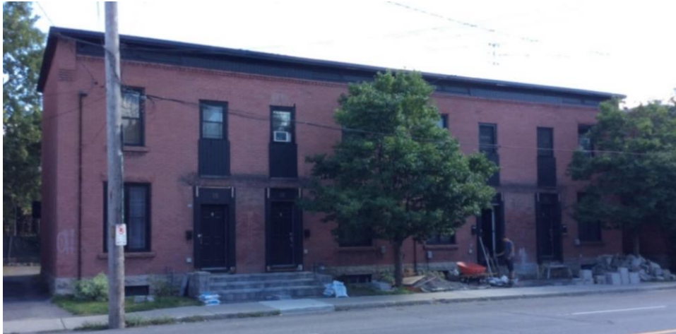
Figure 4: Street view of 12 Hawthorne the subject of this report. The property consists of four townhouses set on 6.m wide lots. The photo dates from circa 2016-2020. The entrance steps are being rebuilt and the existing entrance awnings have yet to be installed. Source: City of Ottawa
