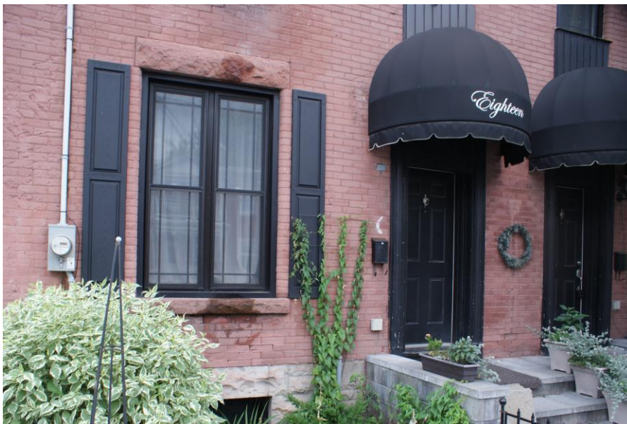
Figure 11: View of the ground floor of one townhouse showing the typical masonry assemblies and detailing. Source: Commonwealth.
