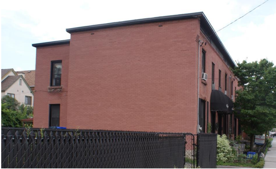
Figure 14: View of the side elevation showing the arrangement of windows on the ends of the row of townhomes. Source: Commonwealth.
