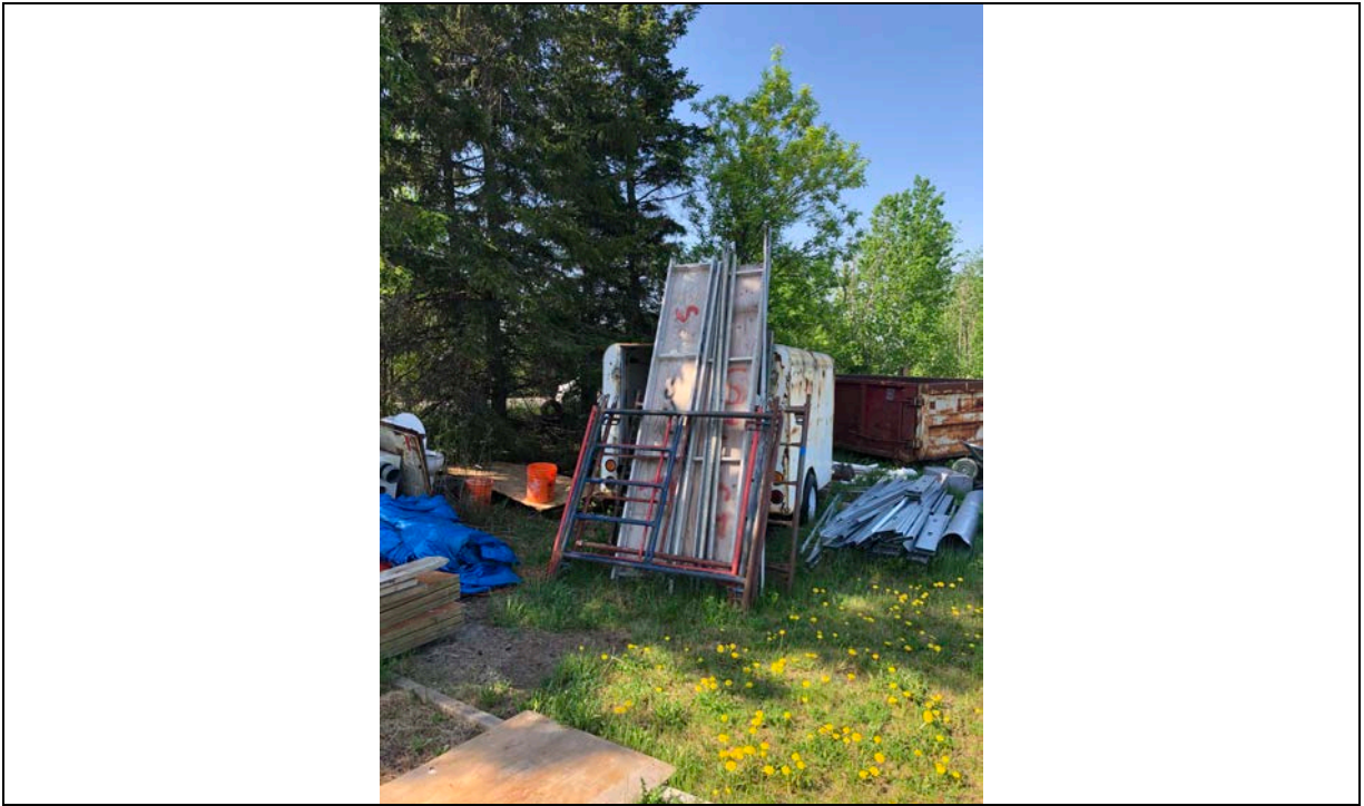
Photo 5 View of construction material in southern portion of the Site.
