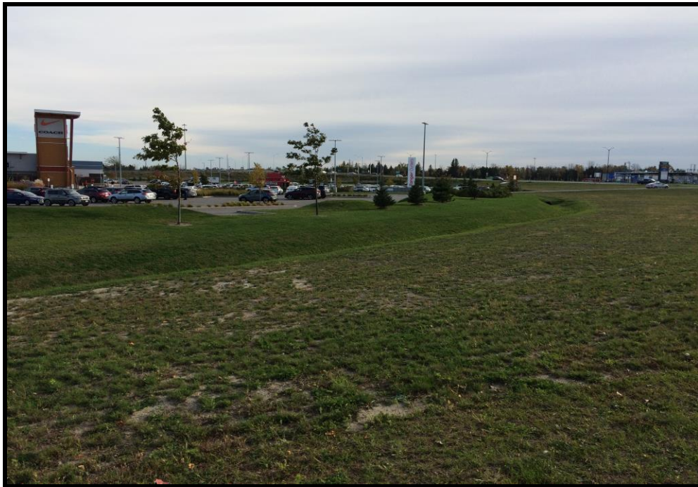
Photograph 4: View of the north portion of the property, as well as an alternate view of a drainage ditch located on the eastern portion of the property, facing south.
