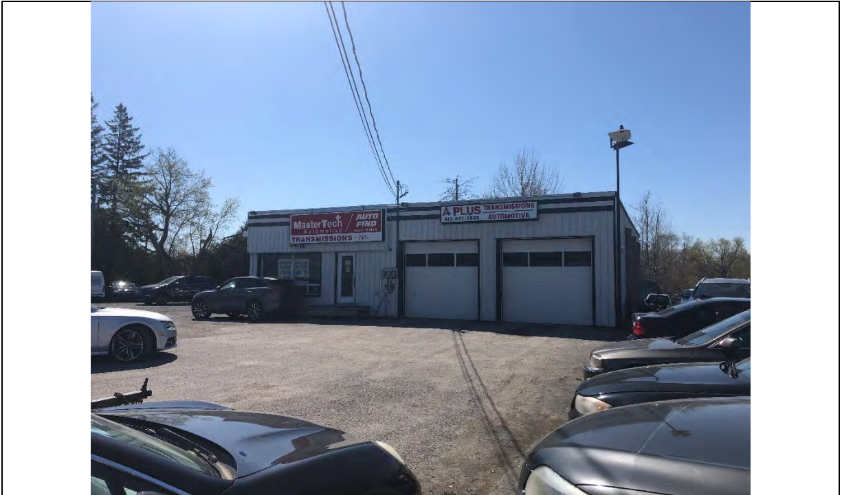
Photo 013 View of MasterTech automotive services located at 3714 Navan Road, south of the Site across Navan Road (facing south).
