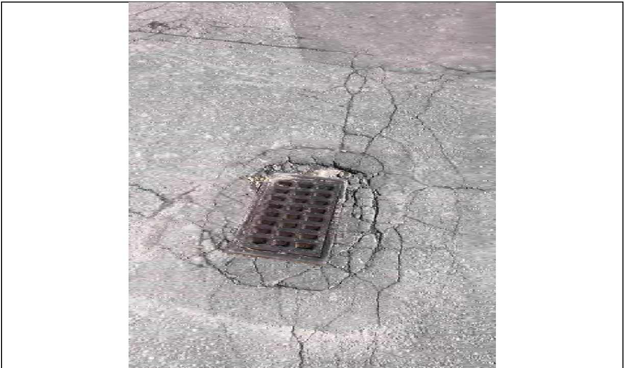
Photo 006 View storm drain in the parking lot on the Site.
