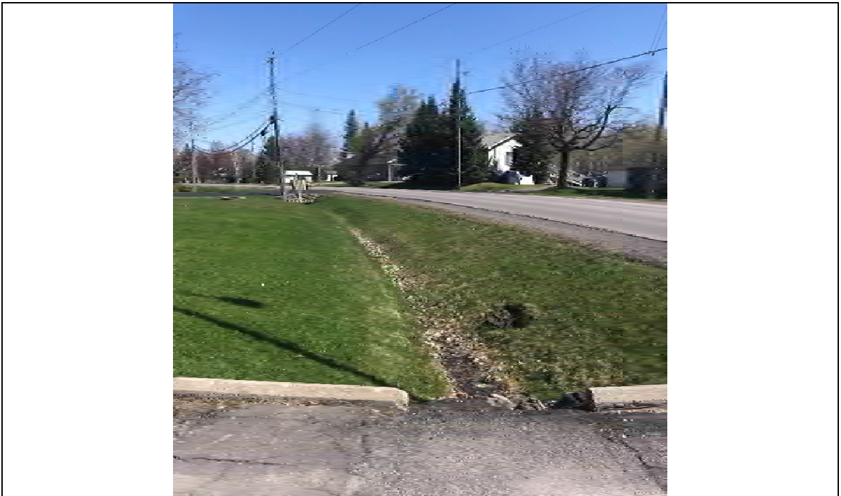
Photo 007 View of the storm ditch along the eastern portion of the Site separating the Site from Mer Bleue Road (facing north).
