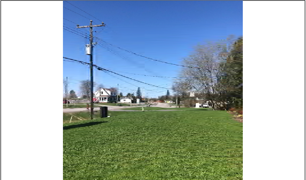
Photo 011 View of pole-mounted transformer and grassy area on the southern portion of the Site where reportedly the septic field or septic holding tank is anticipated to be located (facing west).
