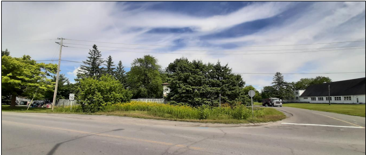
Figure 9: View of Residential Use on Saphir Avenue, East of Mer Bleue Road and the Site
