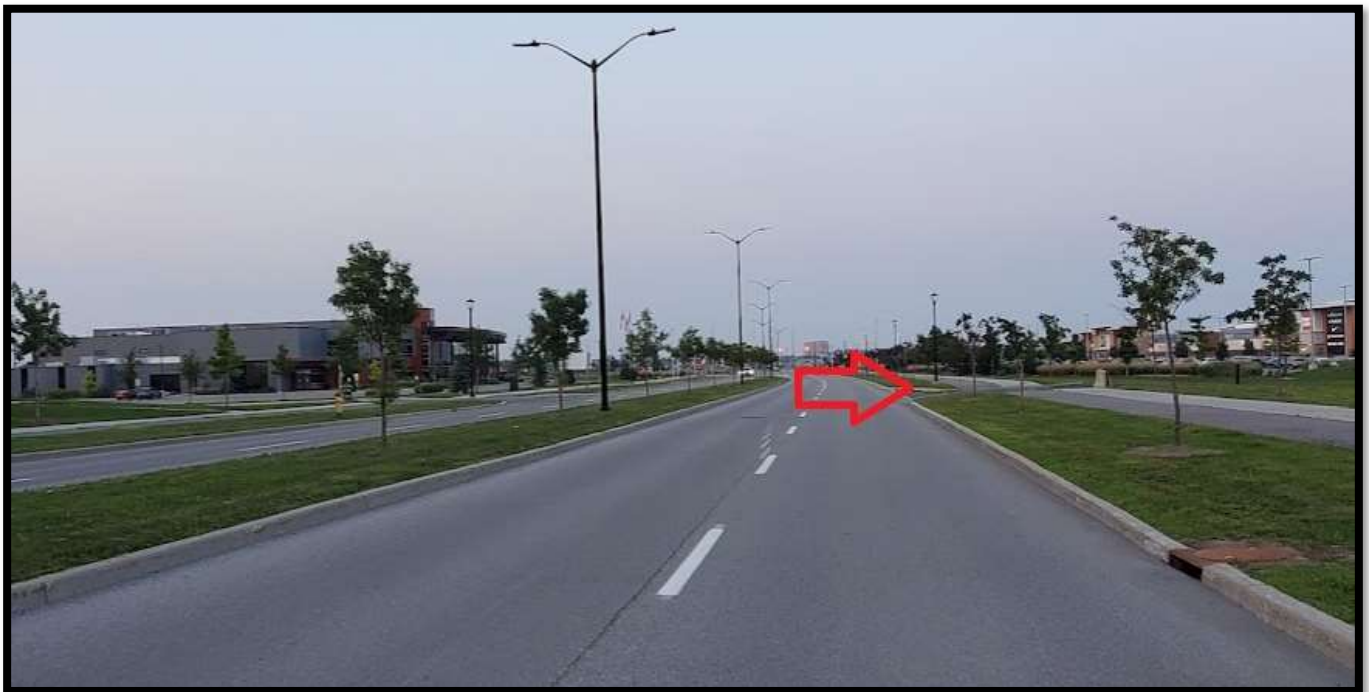
Exhibit J: Facing east on Campeau Drive with the entrance to the Subject Property marked by a red arrow
