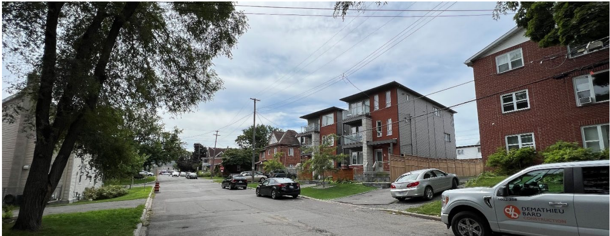
Image 1: Recently Constructed Multi-Unit, Low-rise development along Winona Avenue
