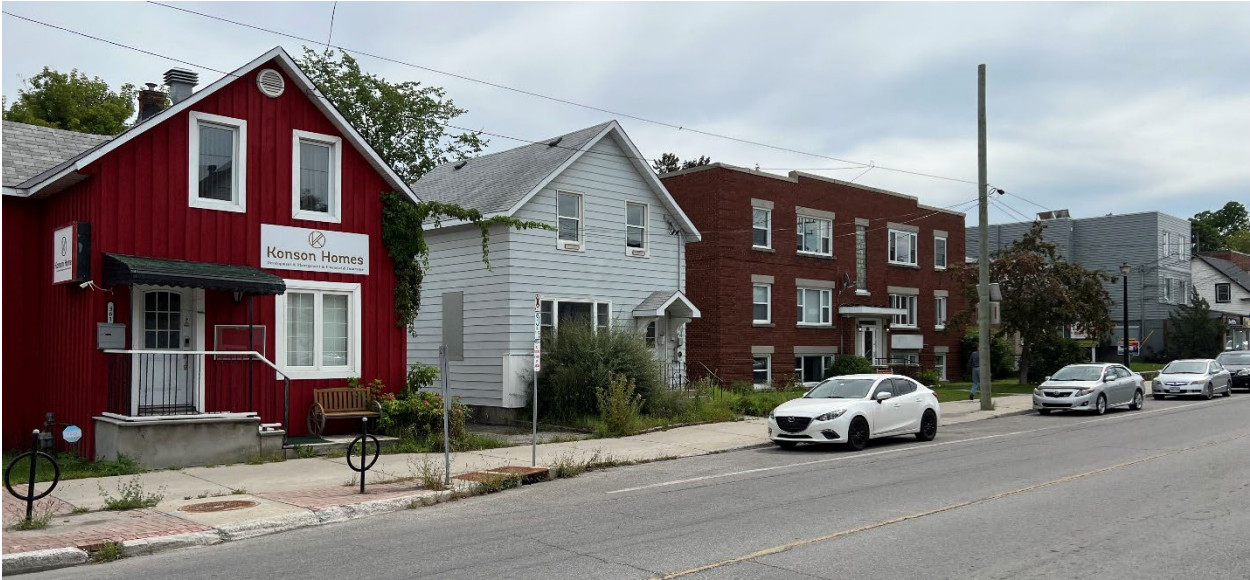
Image 7: Multi-Unit Low-rise development along Churchill Avenue N
