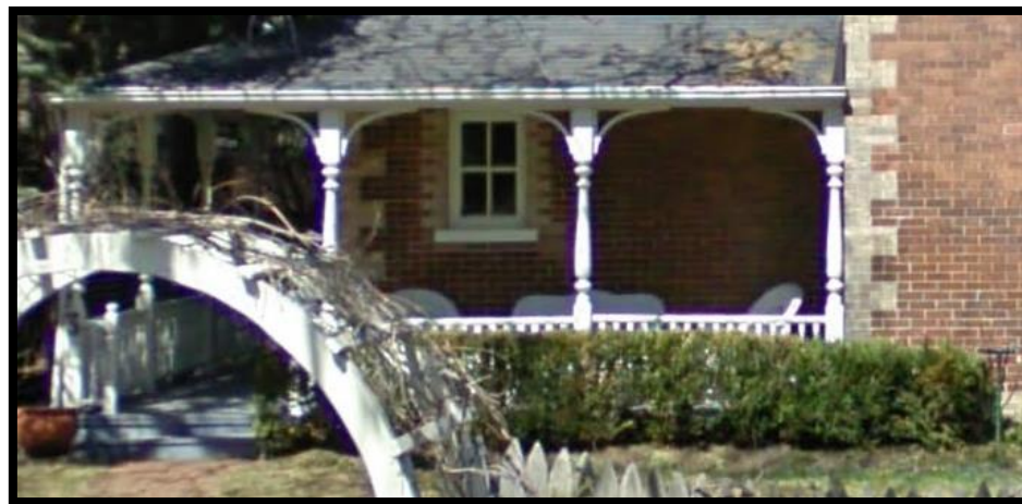
Figure 18: Example of original, or near original posts on the porch of 3 Bower Street, designated by the City of Ottawa as a heritage property in 1978. The house is an exceptional example of Victorian architecture in Ottawa. The woodwork and dichromatic brickwork is representative of Victorian detailing. Credit: Google Streetview; image taken April 2009.
