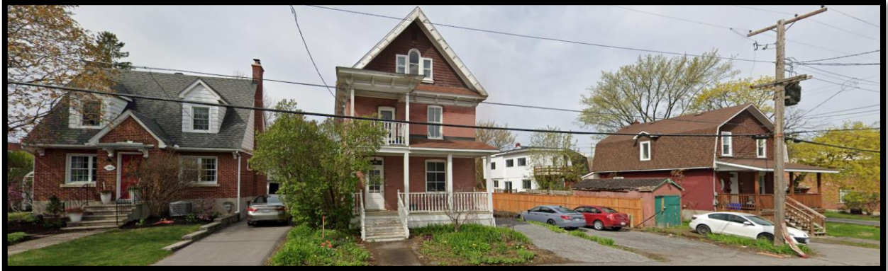
Figure 5: View of 366 Winona Avenue with 368 Winona (left, built c 1950) and 360 Whitby Avenue (right, built c 1920). Credit: Google Streetview, April 2021.
