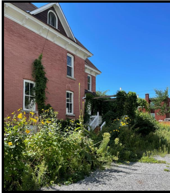
Figure 3: 366 Winona Avenue, 12 August 2022, north elevation, showing the kitchen wing at the rear. Credit: Matrix Heritage.
