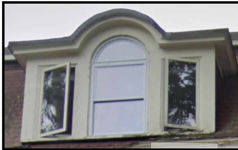
Figure 14: Palladian-inspired dormer window in the attic storey of 730 Echo Drive, a property included on the City of Ottawa Heritage Register. This window features a unifying entablature that includes a curved portion about the curved window. Credit: Google Streetview (detail).
