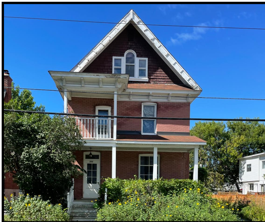
Figure 15: Main elevation of 366 Winona Avenue, showing arrangement of the porch and second-storey portico. The ghosted outline of the original posts for the porch is visible on the brickwork behind the north post. Credit: Matrix Heritage, 2022.
