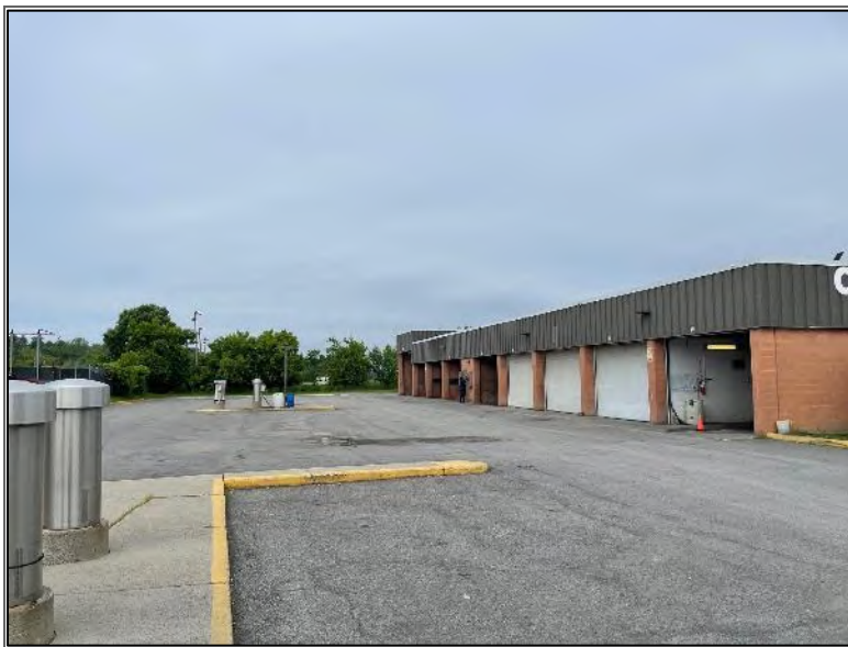
Photo 2 – Site Building (south elevation).
