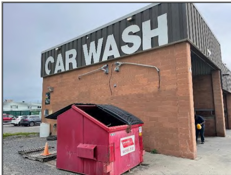
Photo 4 – Site Building (west elevation).
