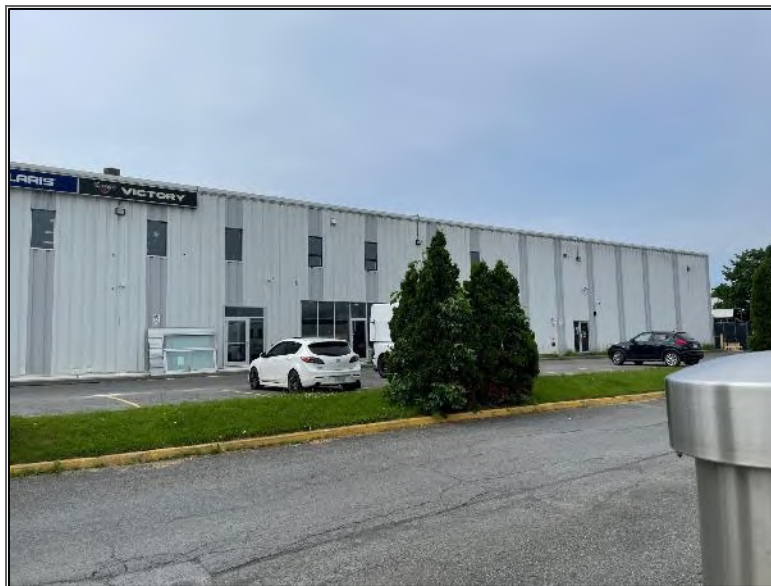
Photo 6 – Property located south of the Phase One Property.
