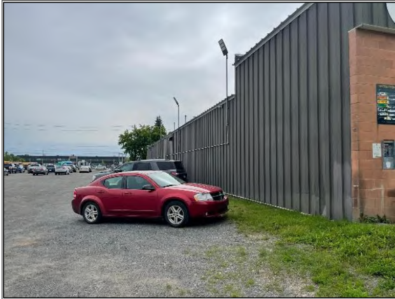
Photo 1 – Site Building (north elevation).
