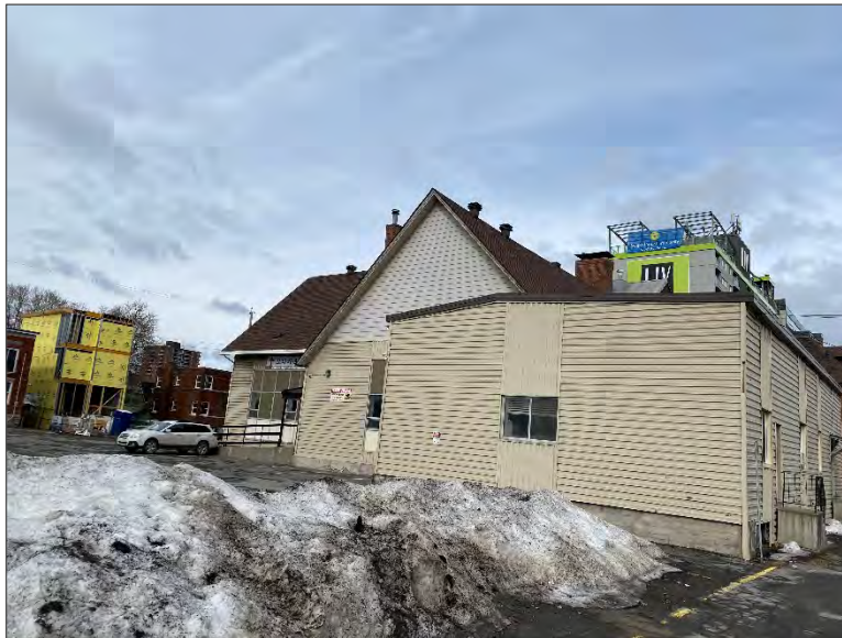
Photo 2 – Site Building (south elevation).
