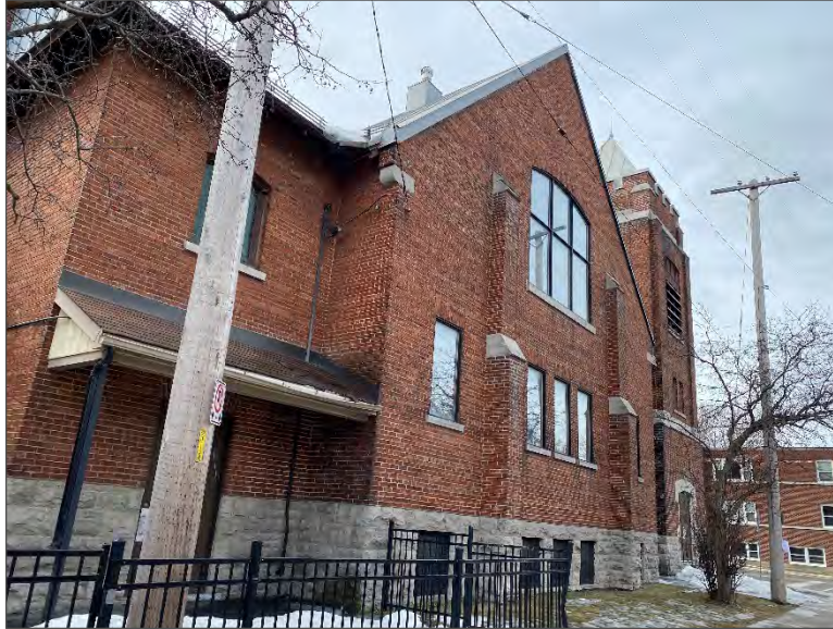
Photo 1 – Site Building (north elevation).
