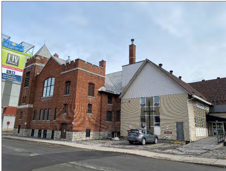
Photo 4 – Site Building (west elevation).
