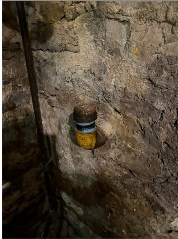
Photo 9 – Pipe indicating the presence of a former AST located in the basement of the Site Building.
