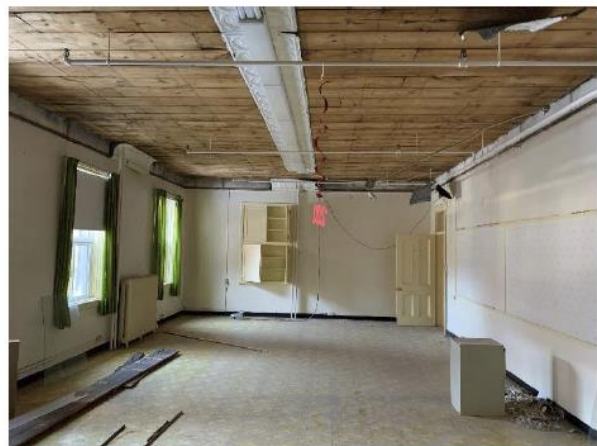
Figure 23: North wing with stripped ceiling finishes
