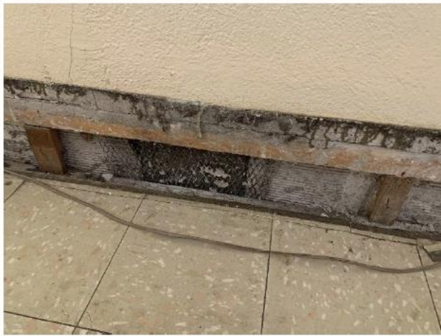
Figure 16: Detail of removed baseboard
