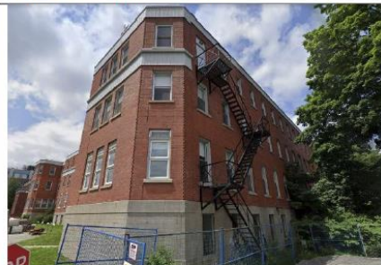
Figure 4: South-East corner of the property from Oblats Ave
