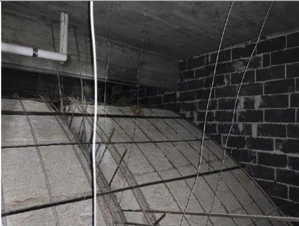
Figure 41: Ceiling cavity. Arch over chancel
