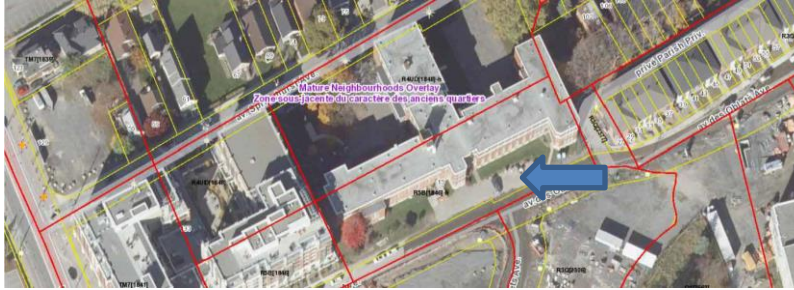
Figure 1: Aerial view illustrating the existing built form and landscape context of the development site – 15 Oblats Avenue. The former Convent is a four-storey brick clad masonry building in a T-plan constructed in four or more phases – 1914, 1926, 1940, and 1954. Building arrowed. Source: Geottawa
