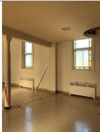
Figure 19: Removed circular stair at chapel
