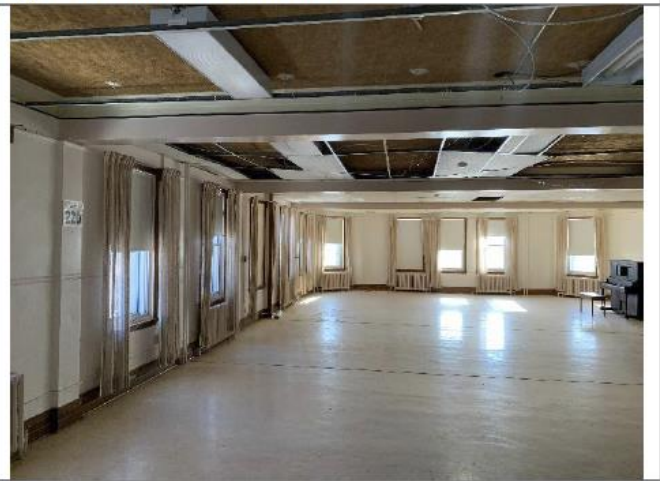
Figure 29: Context of room with ceiling system removed
