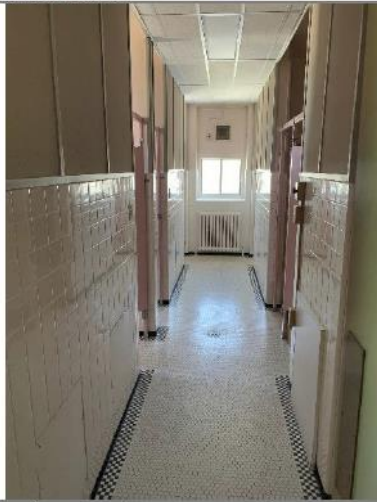
Figure 35: Bathroom Hallway – Women's
