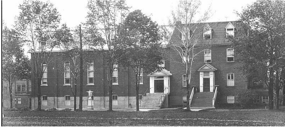
Figure 3: 1926 photograph of the convent. The 1914 structure is to the right and the circa 1926 addition to the left of the image. Note the three-bay form of the 1914 structure, and brick extension for the bell tower to the right. The circa 1926 addition with five window bays with the coloured glass in the sash to the side of the entrance. Note the statue with extended arms in front of the circa 1926 chapel addition. The 1940 chapel extension featured the same brick detailing – pilasters dividing the wall into bays with a stepped brick pattern at the eave. Source: Old Ottawa East website.
