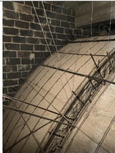
Figure 40: Ceiling cavity. Arch over chancel
