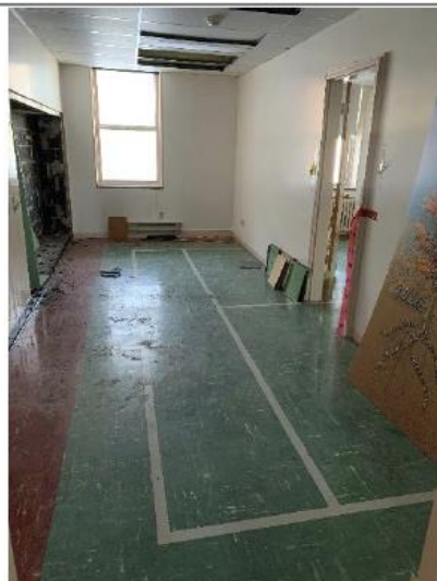
Figure 12: Small modified room with original gymnasium flooring visible
