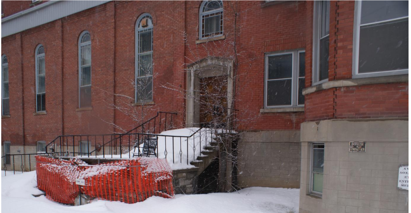
Figure 7: View to the west entrance on the south façade installed circa 1940. Note the round headed windows with the coloured glass in the sash that dates to circa 1926. The entrance and round headed window assemblies are a heritage attribute of the building that will be retained on the south and north facades. Source: Commonwealth
