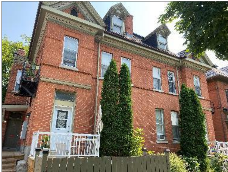
Photo 2 – Site Building (southwest elevation).
