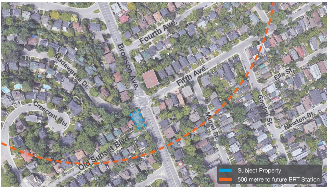
Figure 2: Aerial of subject property, surrounding area, and proximity to future rapid transit.
