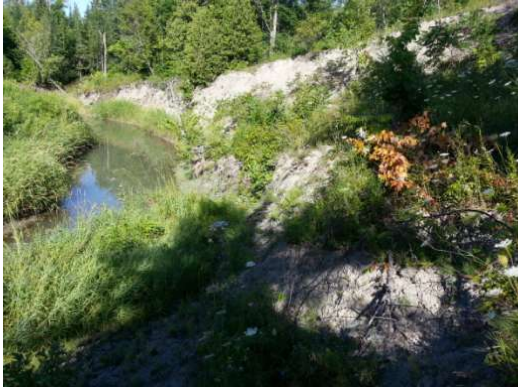
Photo No. 2 – Illustrating the slope failure along the south portion of Slope Cross Section Q on the east slope of Cardinal Creek.
