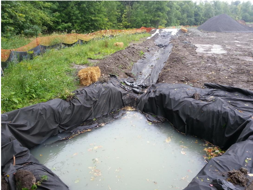
Photograph No. 2 – Photograph of the temporary retention pond 2 (Cell 2) located at the rear of Lots 1 and 2.
