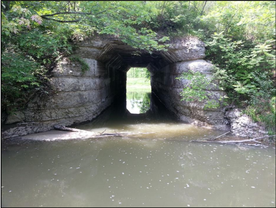
Photo 1 - South face of culvert on July 9, 2013.
