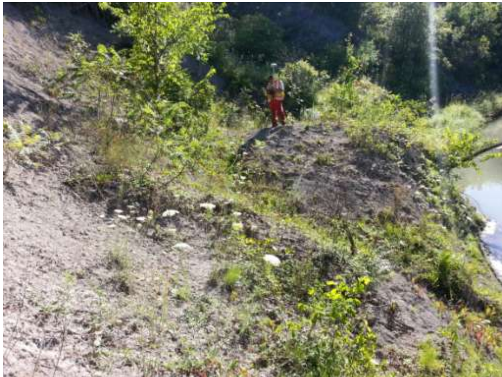
Photo No. 2 – Illustrating the slope failure along the south portion of Slope Cross Section Q on the east slope of Cardinal Creek.
