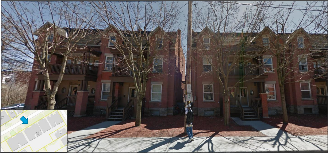
Figure 4: 168 and 166 Osgoode Street front facade.
