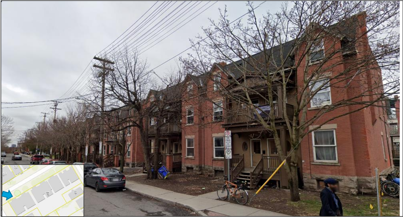
Figure 2: Subject Property, looking east from Nelson Street at 148 through to 168 Osgoode Street.
