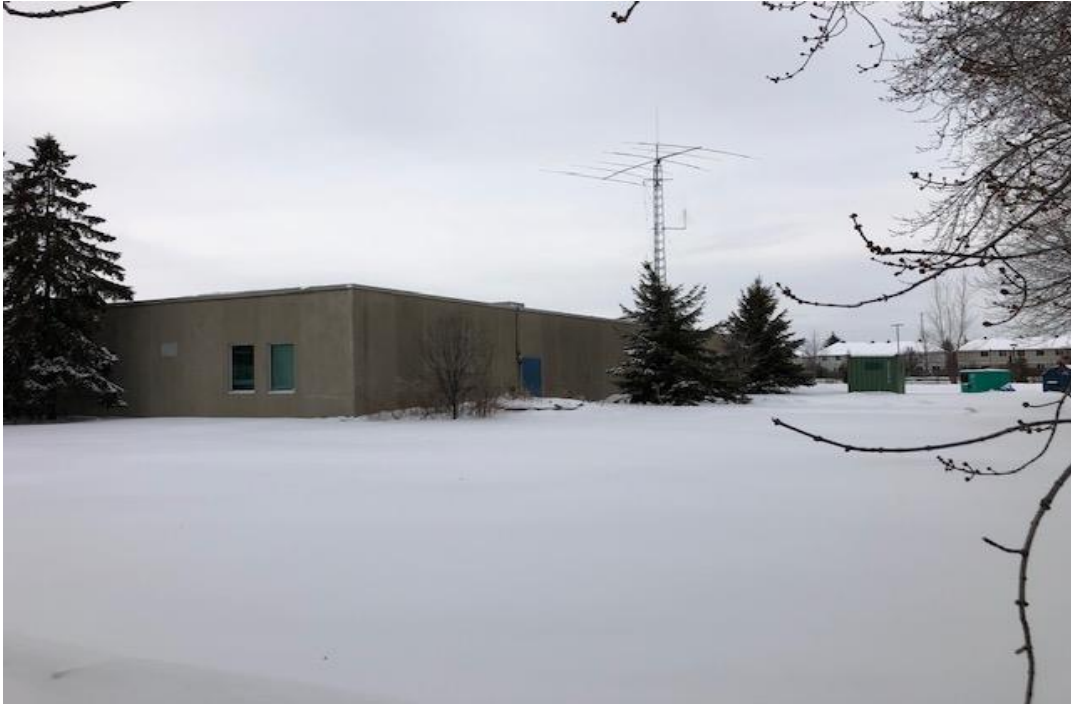
Photograph 3: View of the southeastern portion of the subject site, facing northwest.
