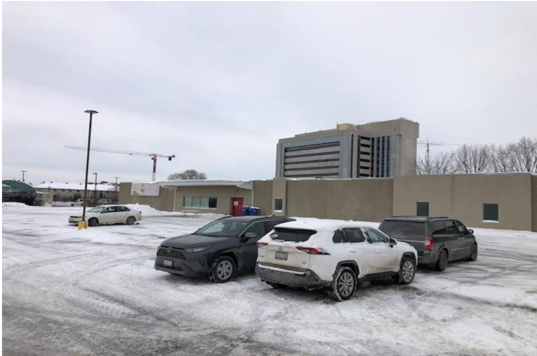
Photograph 1: View of the western portion of the subject site, facing northwest.
