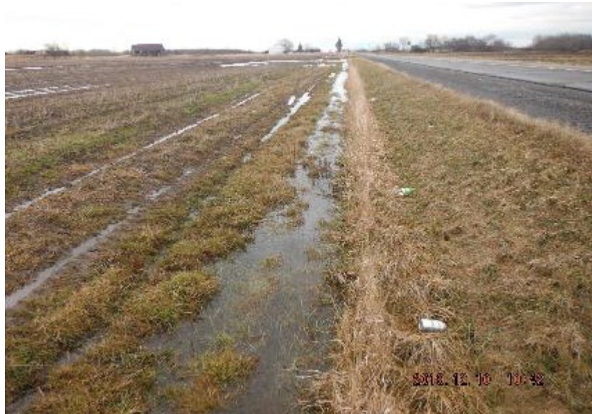
Photo 2: Drain 6 (Station 8) looking upstream from the downstream end (December 10, 2019)
