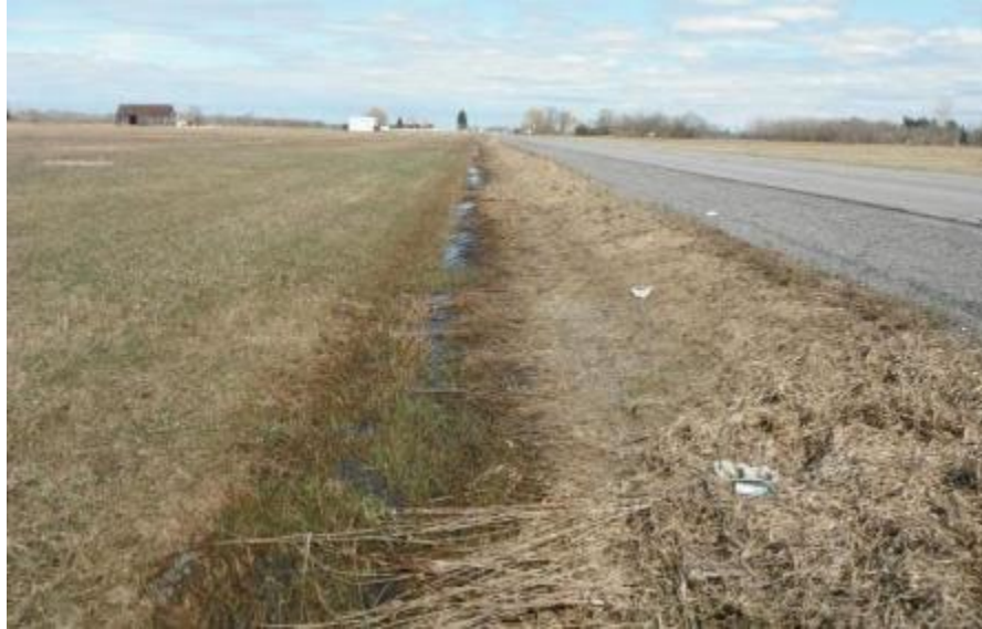
Photo 1: Drain 6 (Station 8) looking upstream from the downstream end (April 28, 2014)
