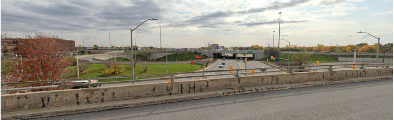
Figure 9: View Looking South from Labelle Street Overpass
