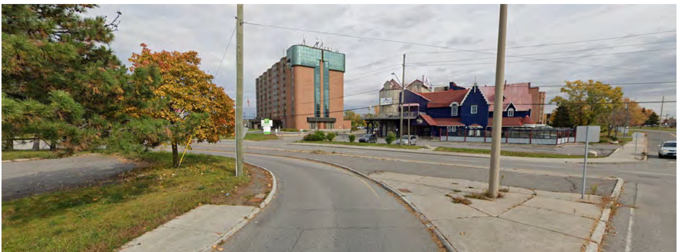
Figure 8: View Looking East from Labelle Street
