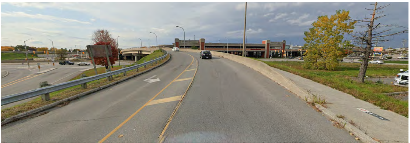
Figure 7: Labelle Street overpass to Transit Station
