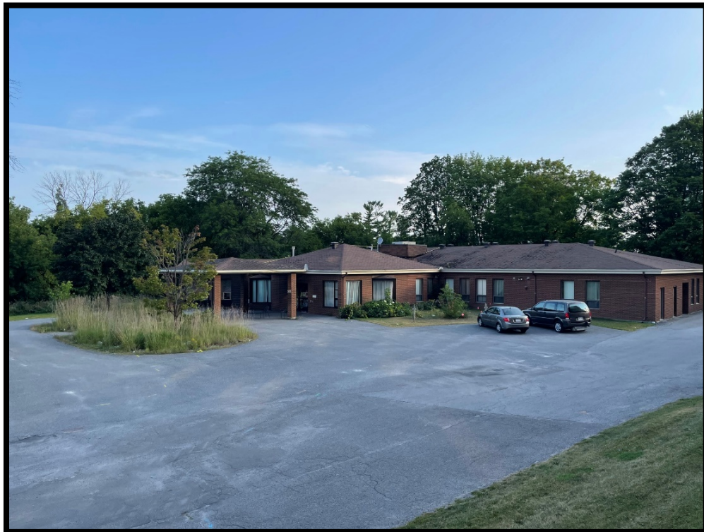
Figure 2: Overview of long-term care facility with parking infrastructure (MH1043-D04).
