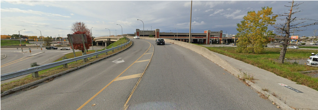
Figure 7: Labelle Street overpass to Transit Station
