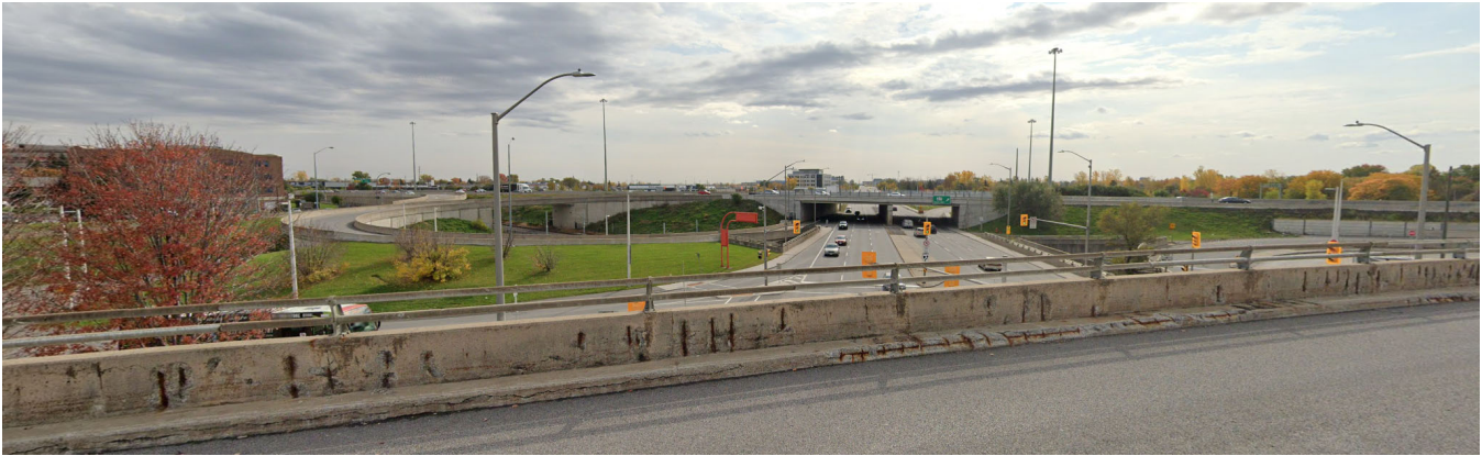
Figure 9: View Looking South from Labelle Street Overpass
