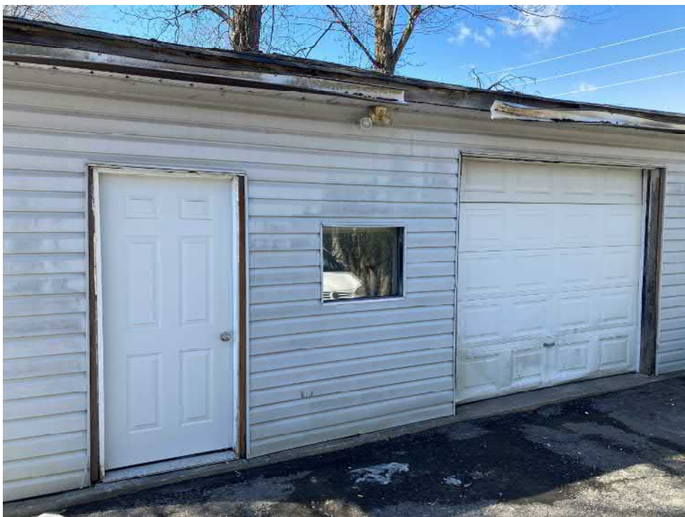
Photo 8: Detached garage, facing west
