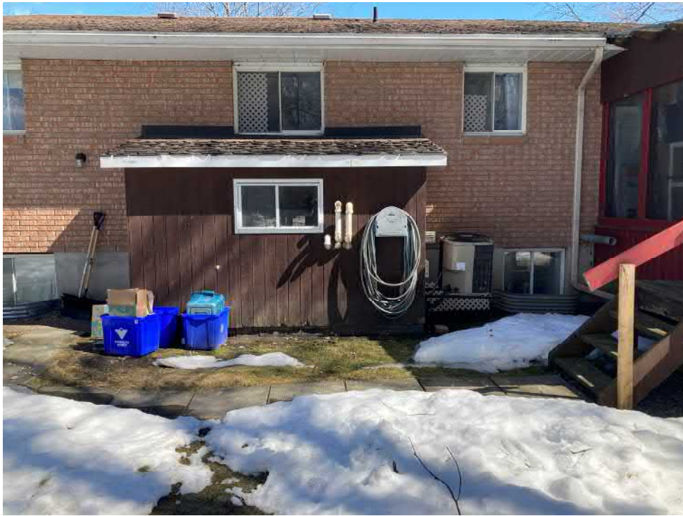
Photo 7: West side (rear) of house, facing east, showing central air conditioning unit and gas furnace exhaust
