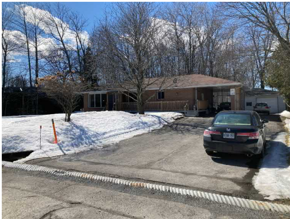
Photo 4: House and driveway, facing east from White Street, showing ditch and corrugated steel pipe culvert along White Street in foreground
