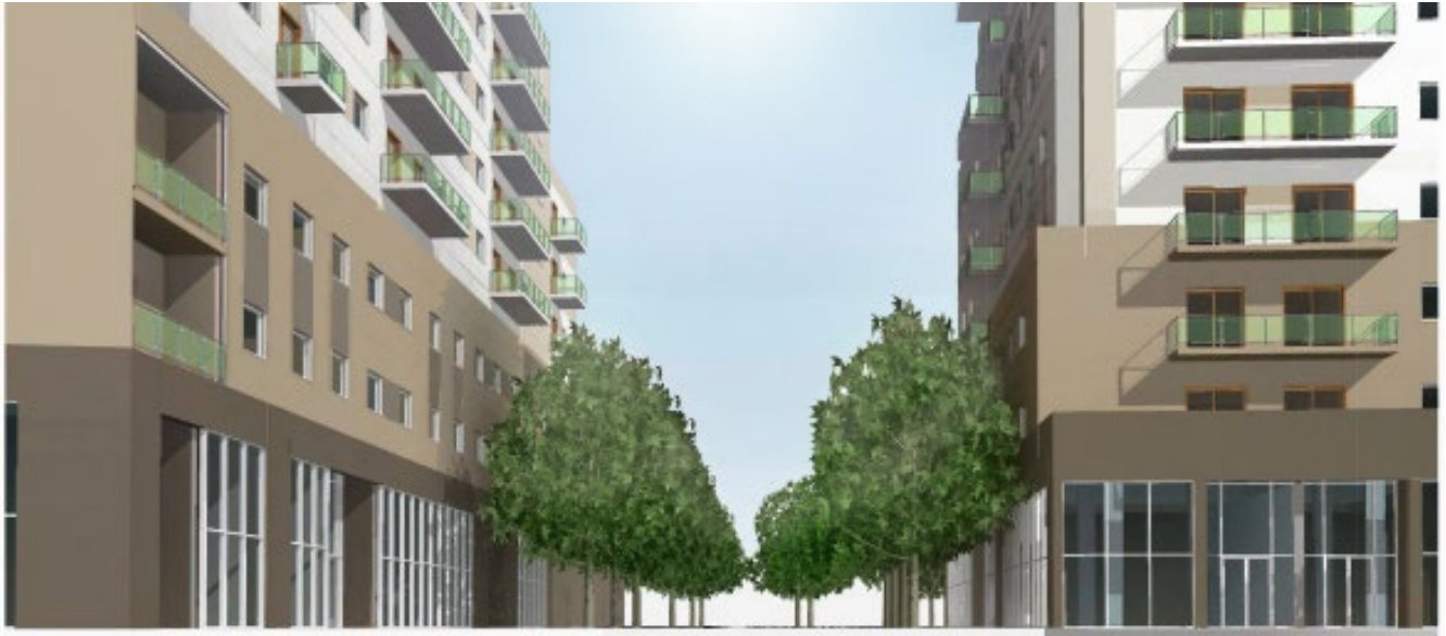
Figure 13. View looking southeast at the subject property from the Hazeldean Road intersection
