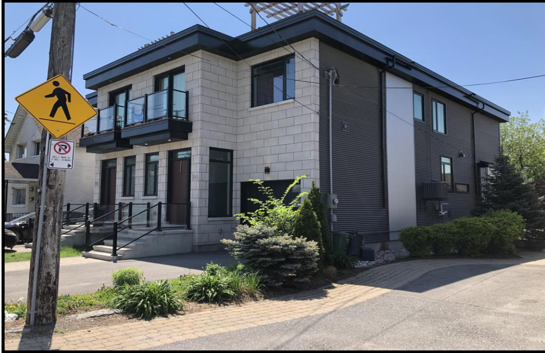
Photograph 1: View of the semi-detached residential dwelling at 318 Athlone Avenue, facing southwest from Athlone Avenue.
