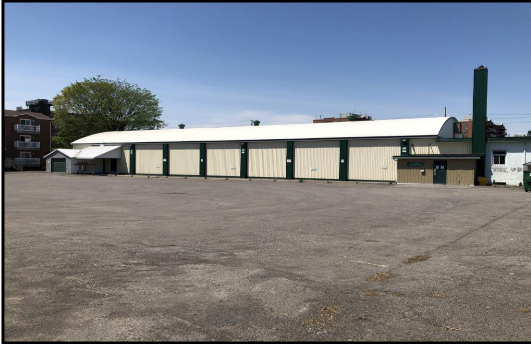
Photograph 5: View of the curling arena at 2026 Scott Street, facing north from Ashton Avenue.
