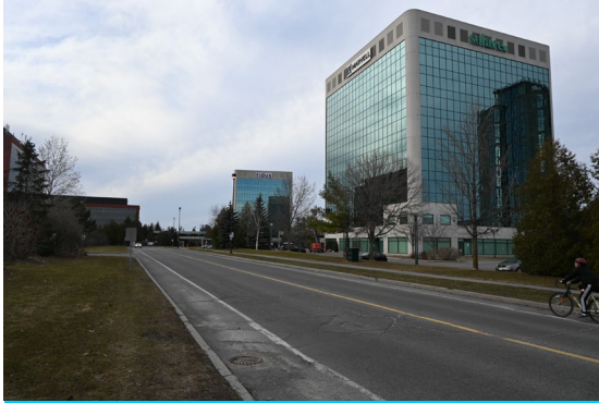
1. Commercial uses on North side of Legget Dr.
