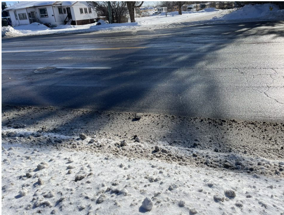
Photo 20 - Manholes on Innes Road
