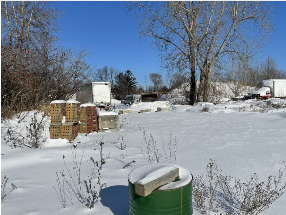
Photo 27 - Stockpiled building material on the Site
