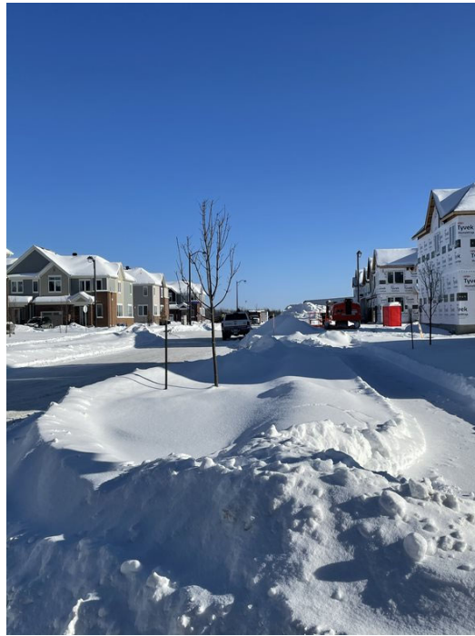
Photo 1 - Active construction off of Lamarche Avenue
