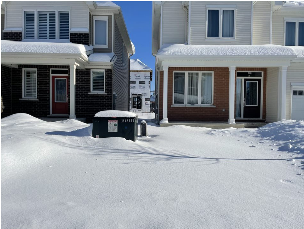
Photo 32 - Utility Box located on Lamarche Avenue
