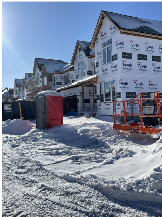
Photo 2 - Active construction site (including temporary hydraulic lift)
