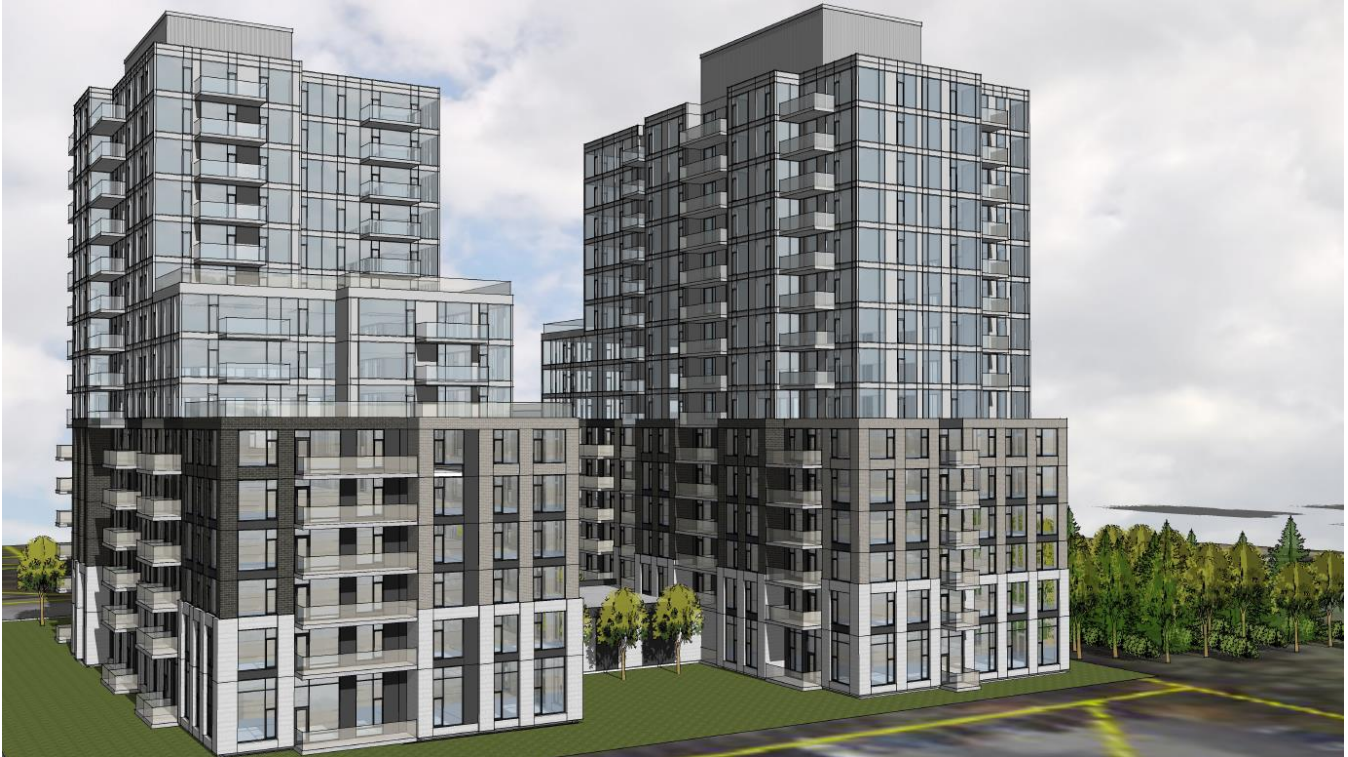
Figure 10: View looking south-east towards the subject site
