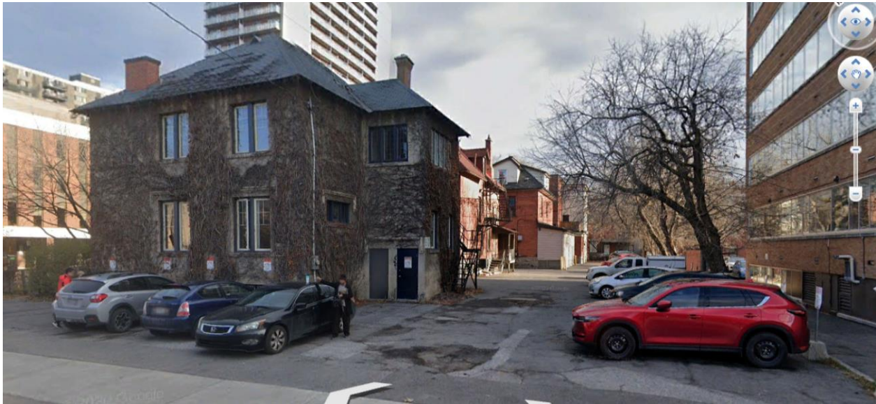
Figure 4: Street view of the side yard of 444 MacLaren and the existing building at 359 Kent (right). The proposed development includes a link that extends to the rear of the buildings at 436, and 444 MacLaren that will provide a secondary access to the new development. Source: Google Earth
