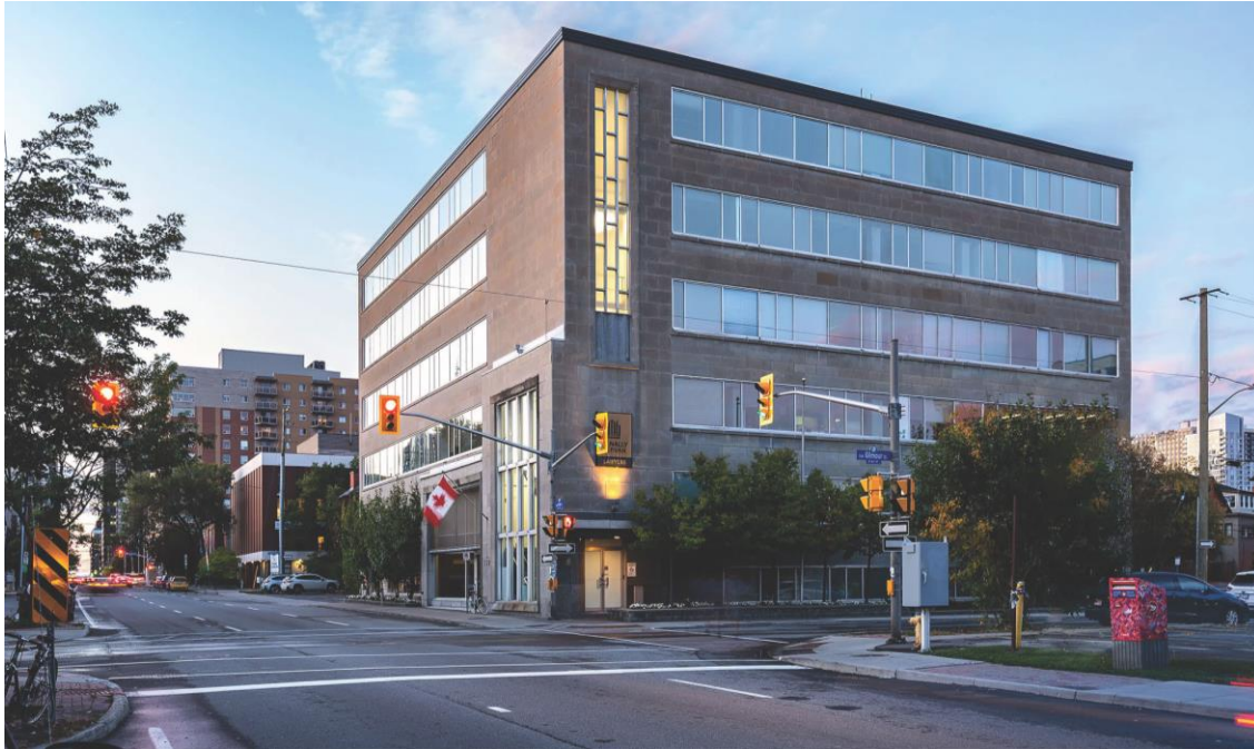
Figure 10: Contemporary view of the Legion House looking north on Kent. Source: Regional Realty
