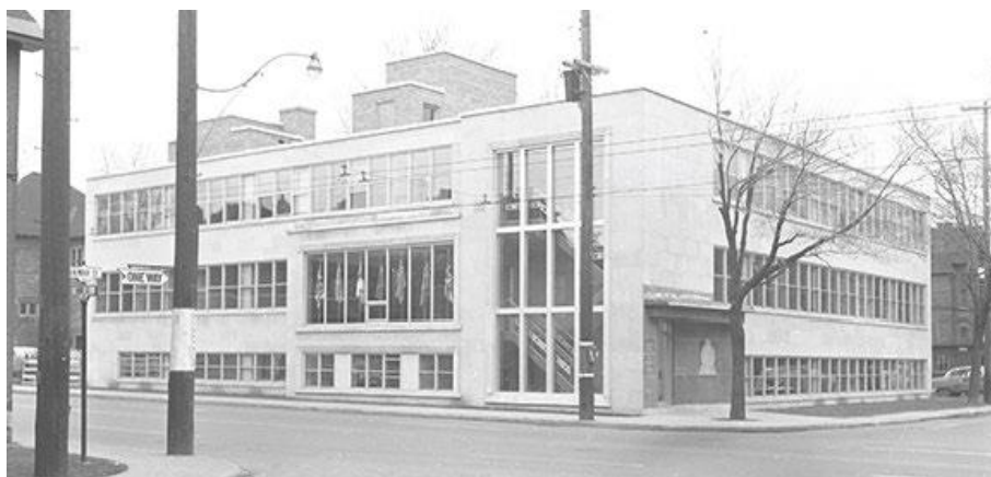
Figure 1: November 1956 photo of the recently completed national headquarters of the Royal Canadian Legion. The entrance was originally off Gilmour Street (right) with a two- and one-half storey glazed window denoting the vertical circulation with a one-storey bay window to the left denoting the publicly accessible portions of the building. Source: Ottawa Archives November 1956
