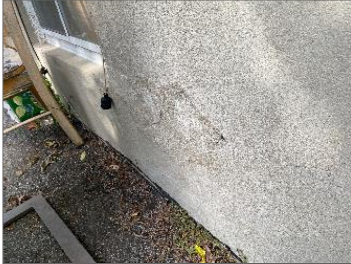
Photo 9 – Patching, inferred to be for a former heating oil AST, observed along the exterior elevation of Site Building B.
