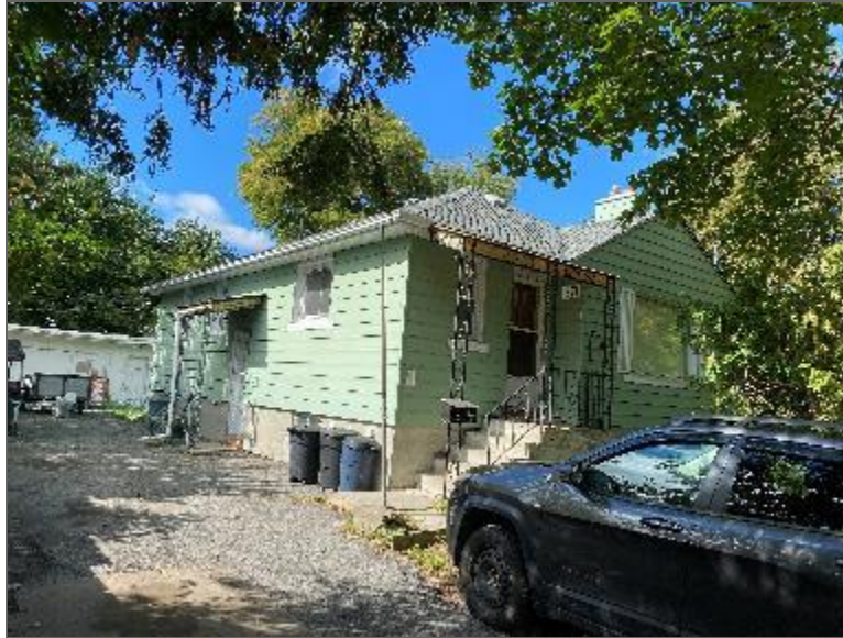
Photo 3 – Site Building B (northeast and southeast elevations).
