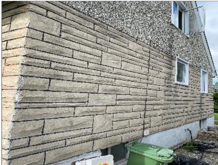
Photo 6 – Site Building C (northeast elevation).
