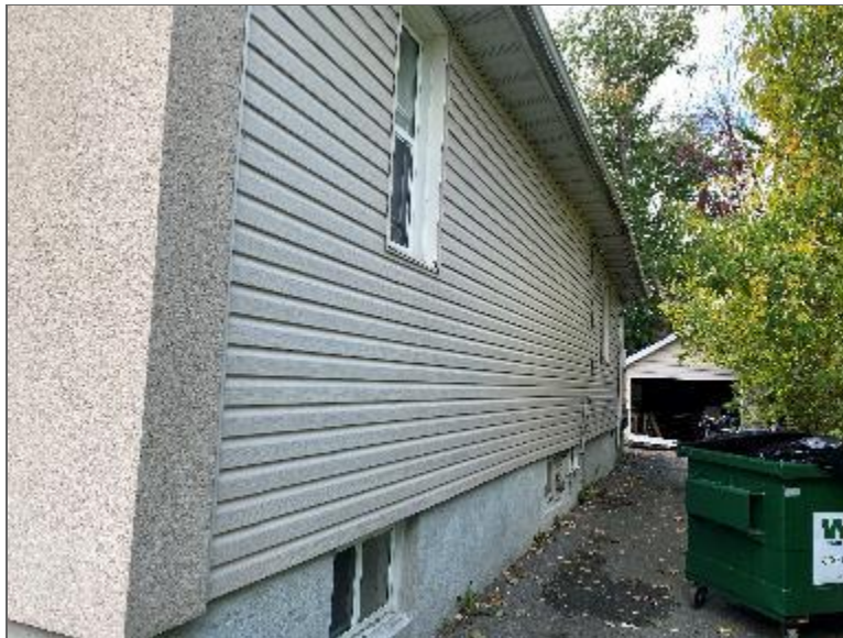
Photo 2 – Site Building A (northwest elevation).
