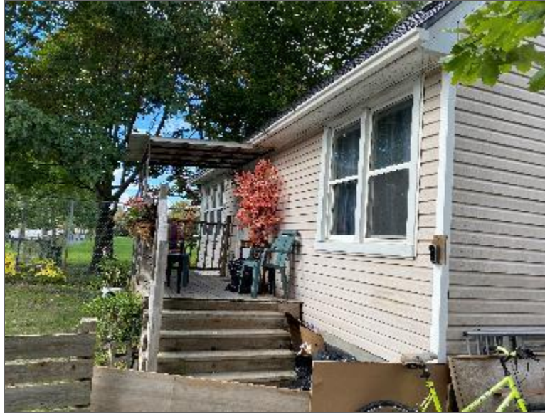
Photo 7 – Site Building D (southeast elevation).
