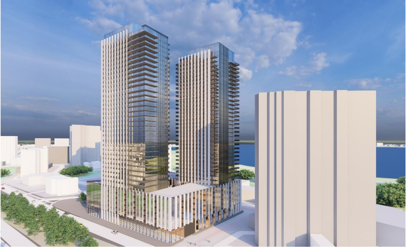
Figure 10: Looking northwest towards the subject site
