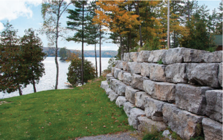
THE PROPOSED BOULDER TYPE RETAINING WALLS ARE MORE THAN 60CM (2 FEET) AND, THEREFORE CAN BE USED AS A TUTRLE BARRIER.
