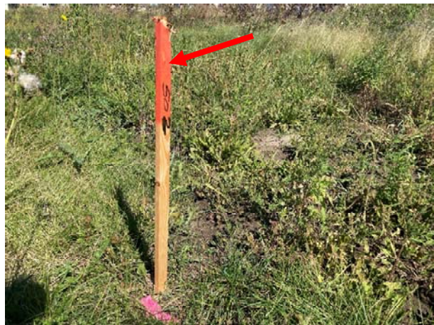
Photo 8. View of the marked buried Hydro One electrical utility line (see arrow) observed adjacent to the west portion of the Phase One Property.
