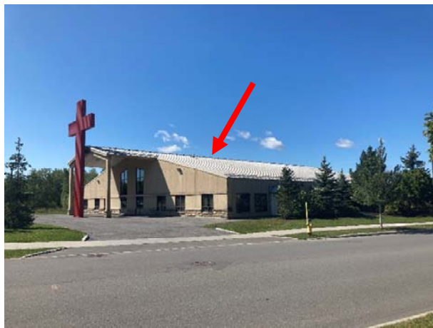
Photo 15. View of the neighbouring property to the west (across Famille-Laporte Avenue) at 1123 Old Montreal Road (see arrow), looking northwest from across Famille-Laporte Avenue.
