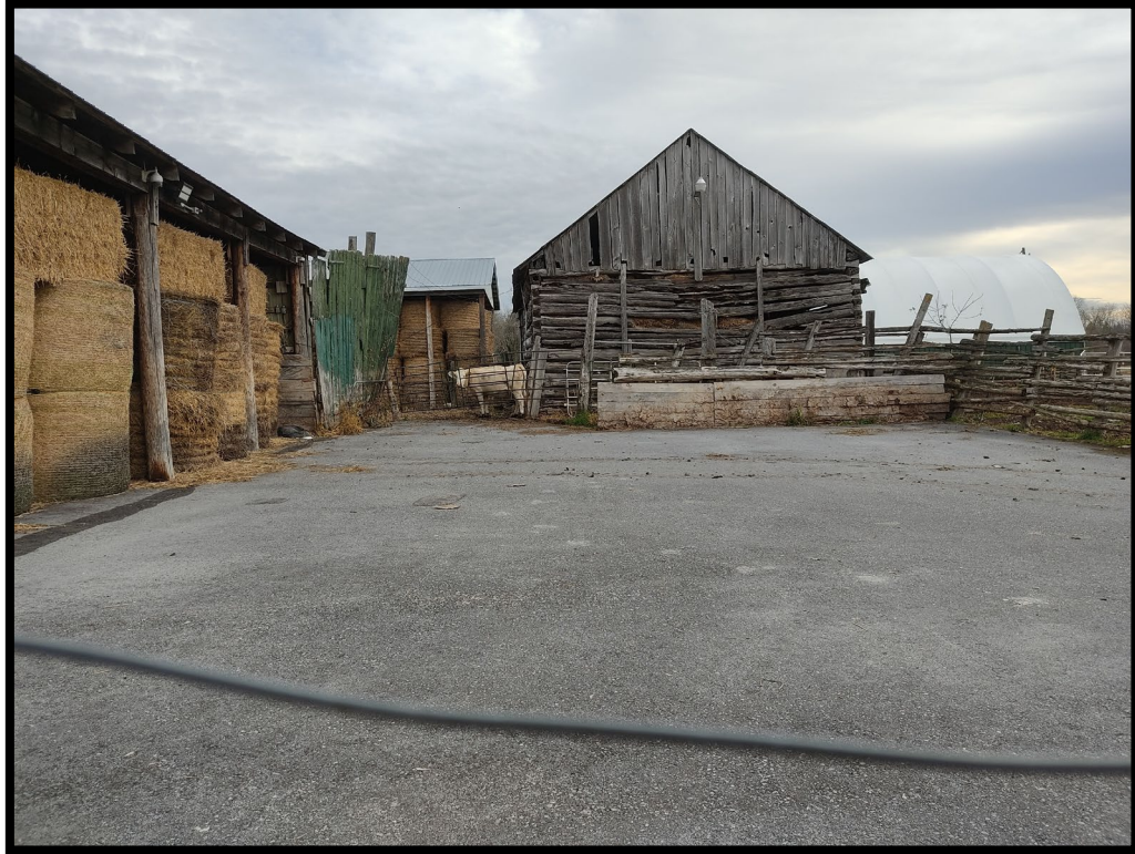
Figure 13: Gravel pad near farm buildings (PA1214-D43).
