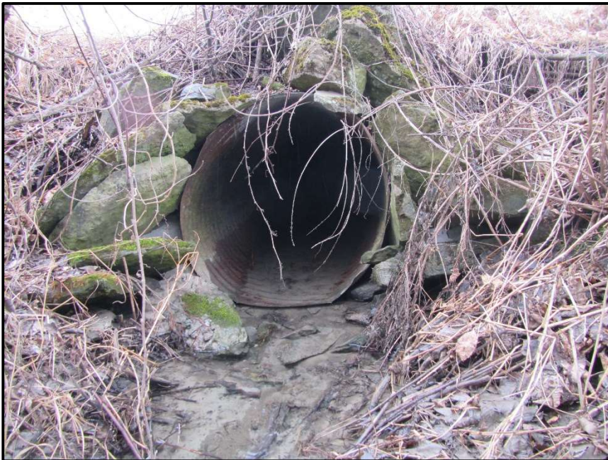
Photograph 6: 850 mm CSP culvert between the upstream and downstream portions of Survey Site #3 (March 24 th , 2021).
