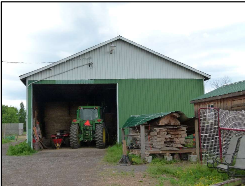
Photograph 18: Structure #2 (Tractor Garage). Two (2) active Barn Swallow nests were observed within Structure #2 (July 29 th , 2020).
