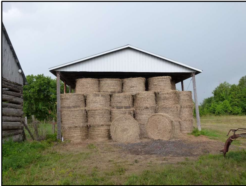
Photograph 25: Structure #6 (Open Hay Storage Area). No Barn Swallow nests were observed within Structure #6 (July 29 th , 2020).
