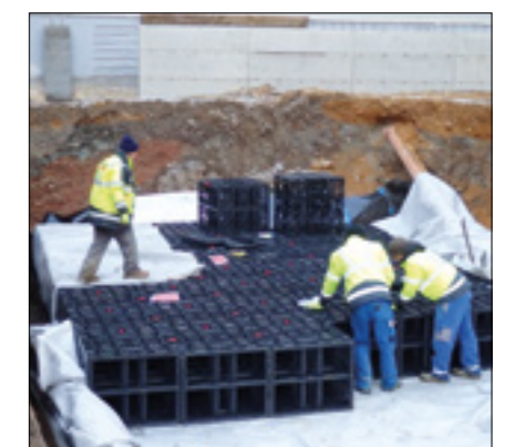
Industrial building, Tumeltsham (AT)
