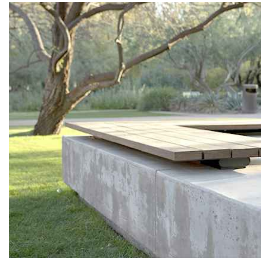
COMMON GARDEN SMALL RETAINING WALL
