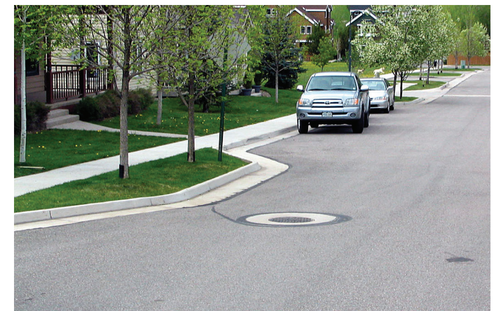
Figure 54 Pinchpoint (Chicane / Curb Extension) Example
