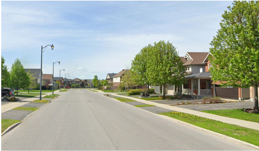
Figure 40 Local (Typical 20.0m Right-of-Way) Example
