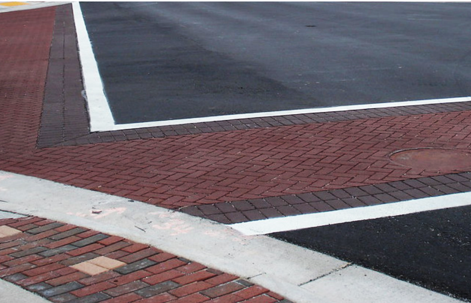
Enhanced Intersection Paving
