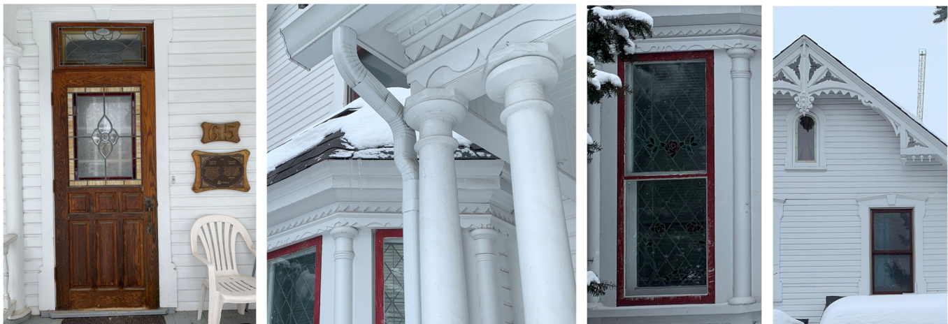
Figure 7: Various exterior notable design features
