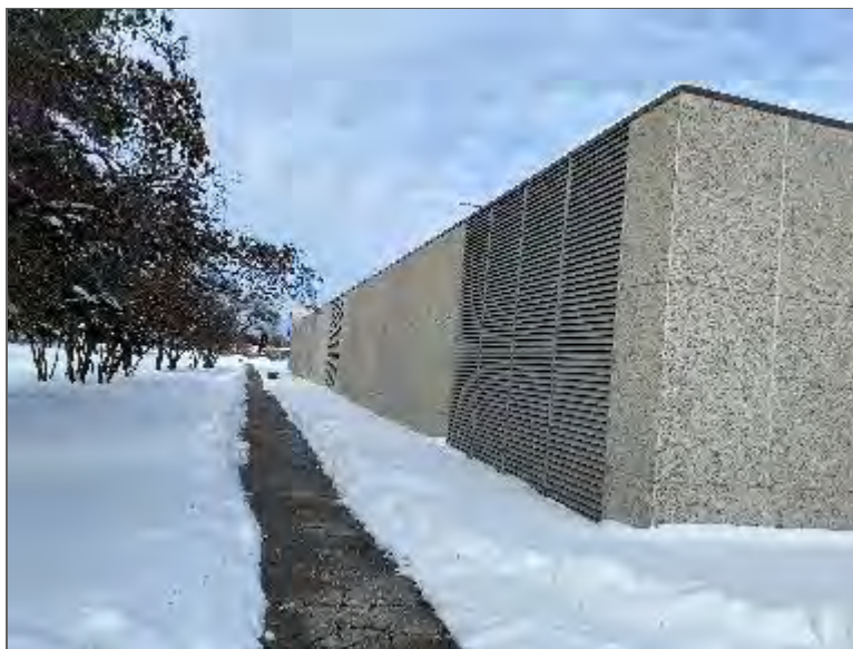
Photo 2 – Site Building A (west elevation).
