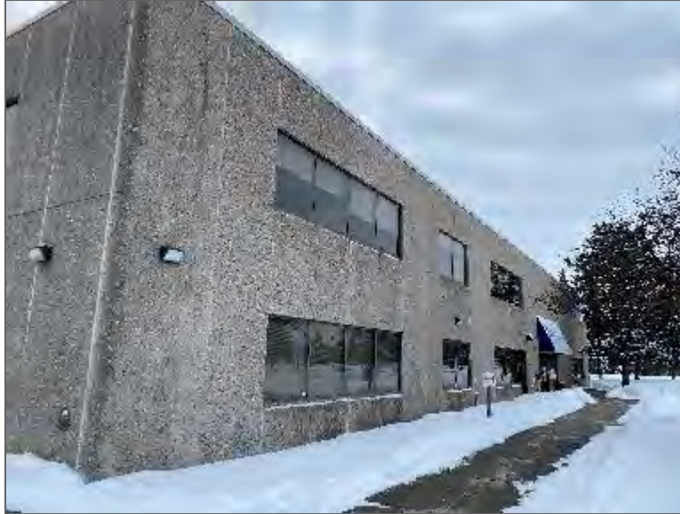
Photo 3 – Site Building B (north elevation).
