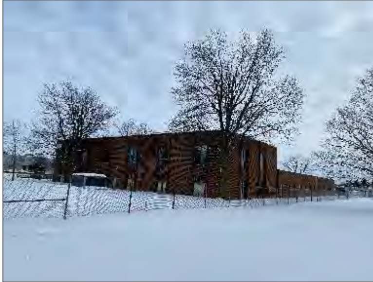
Photo 9 – Properties located east of the Phase One Property.
