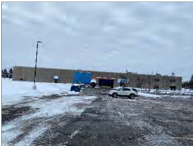
Photo 4 – Site Building B (east elevation).
