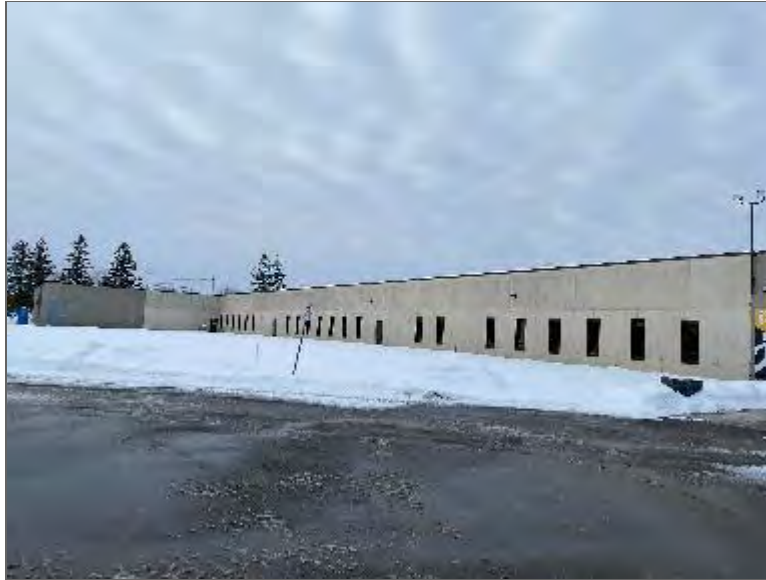
Photo 1 – Site Building A (south elevation).
