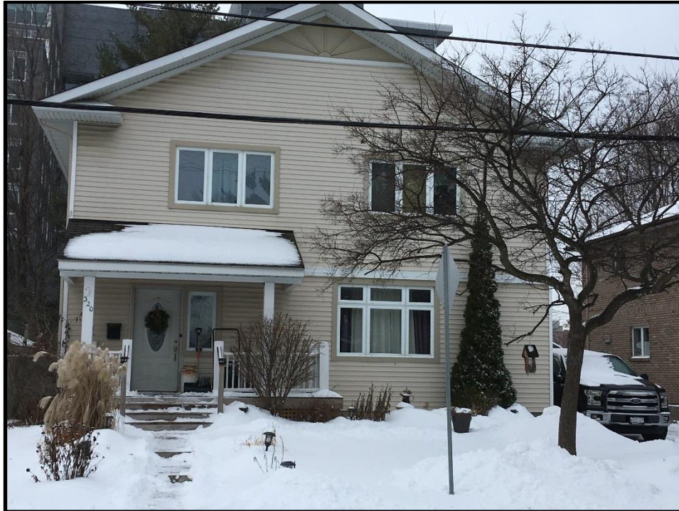
Photograph 2: East face of subject building addressed 320 Clifton Road, looking west.
