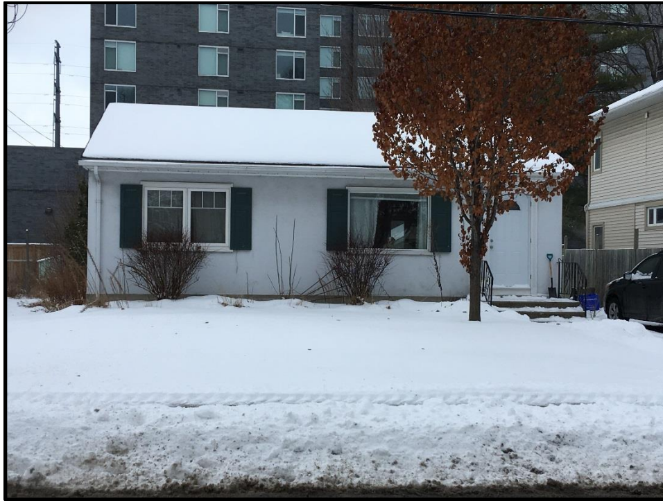
Photograph 3: East face of subject building addressed 324 Clifton Road, looking west.
