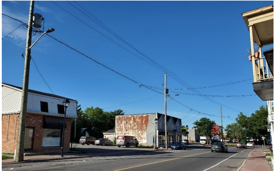
10 Western portion of the subject site on Beechwood Avenue. MTBA
