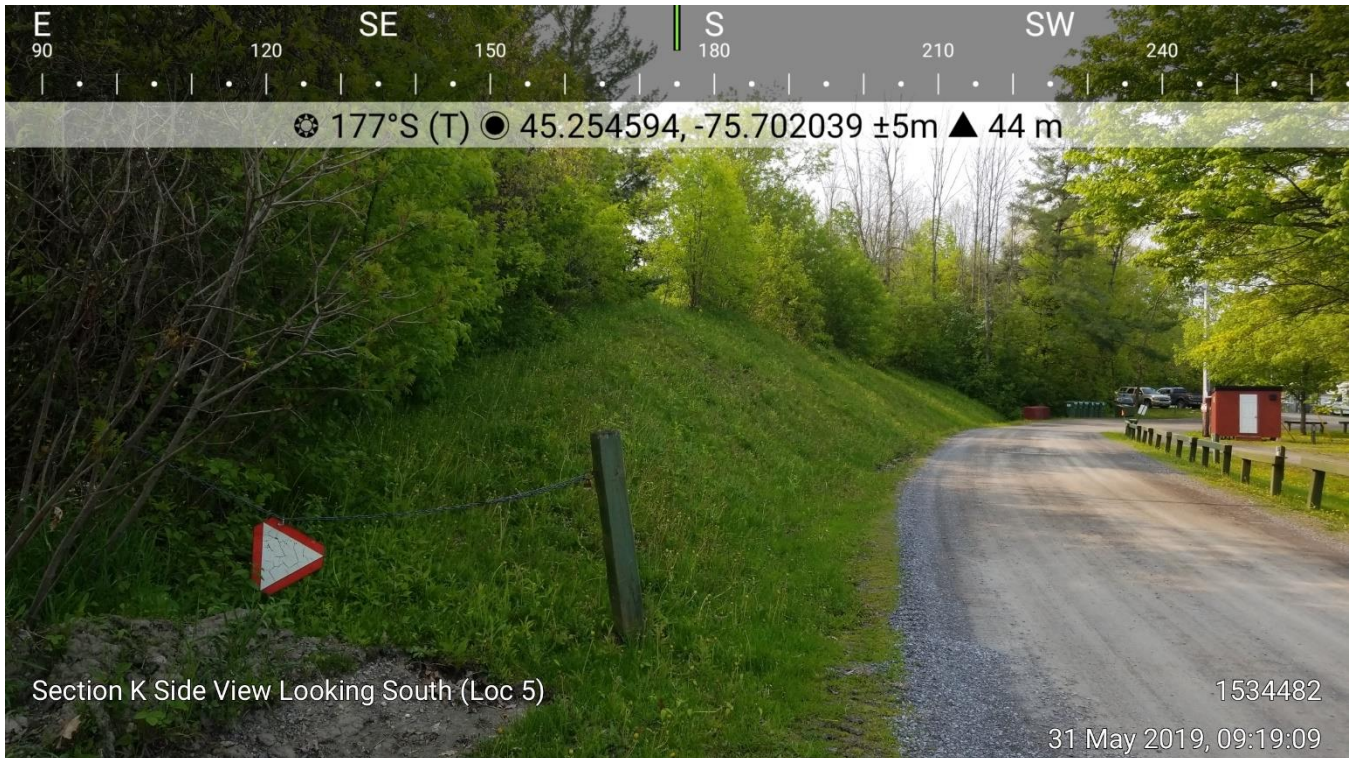
Photo D-12: Western Slopes; cross-section K-K'; looking toward south
