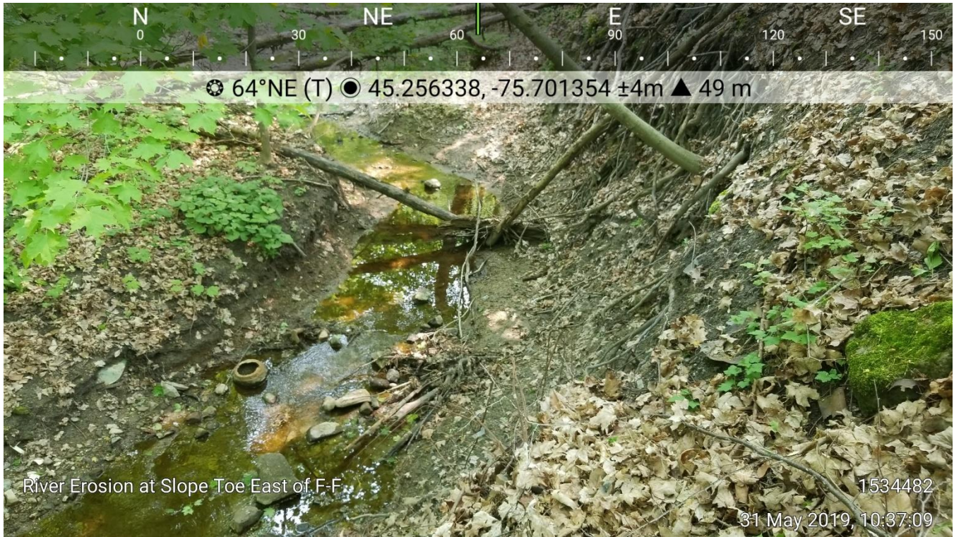
Photo D-7: Northern Slopes; cross-section F-F'; looking toward east
