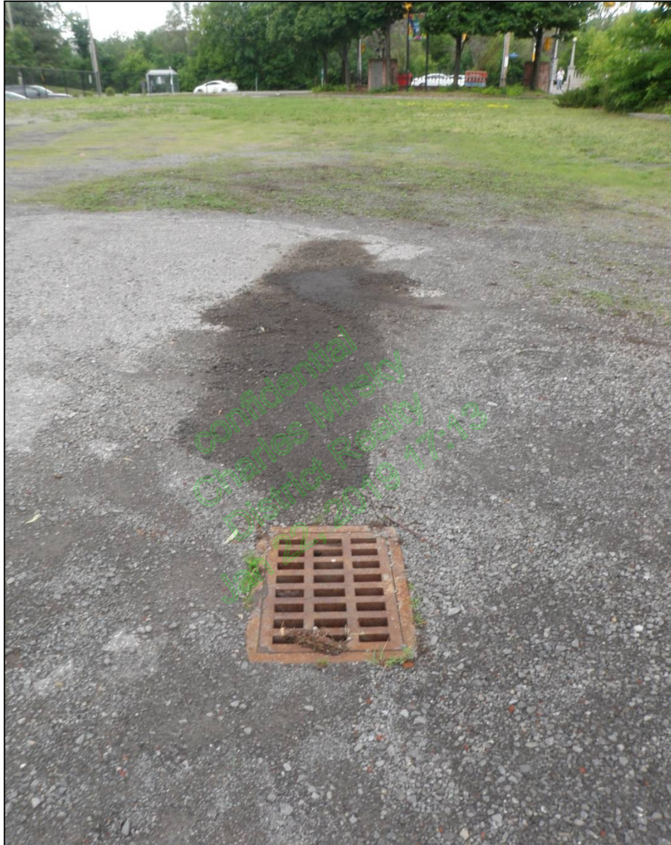
PHOTO 5: Surface staining near catch basin on-Site.
