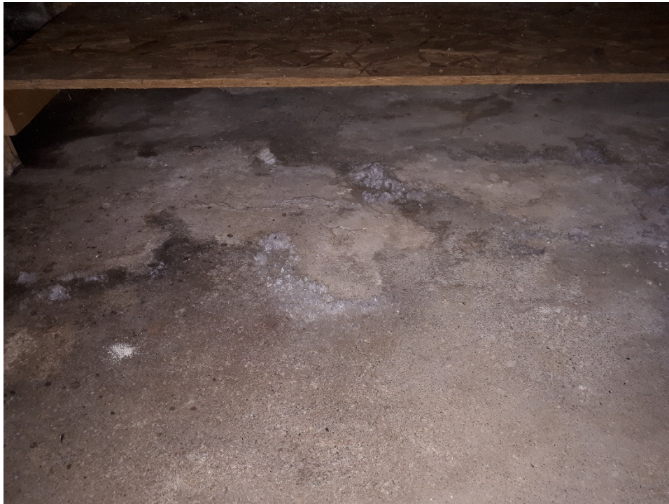
Photo 8: Effluence noted in basement of 252 Hinchey Avenue.
