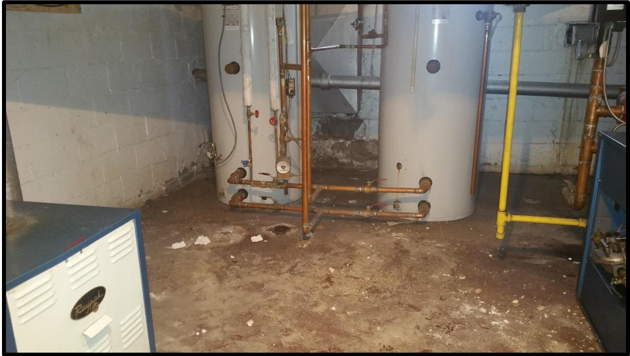
Photograph 7: View of the natural gas fired hot water tanks and boilers within the utility room located in the basement of the eastern motel structure.
